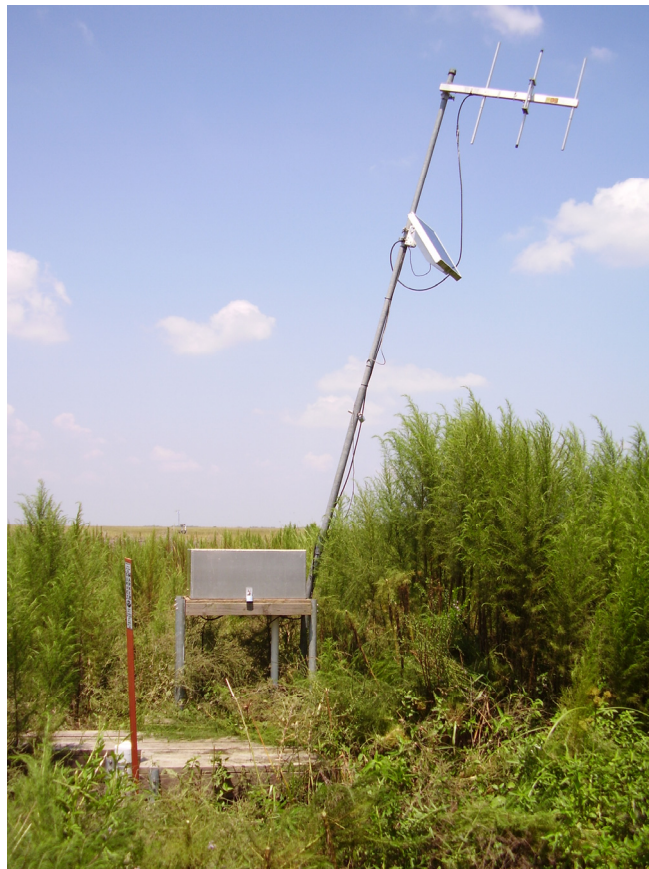
Figure 12: Well cluster 3AN1-GW-4B (on island; view looking east)
