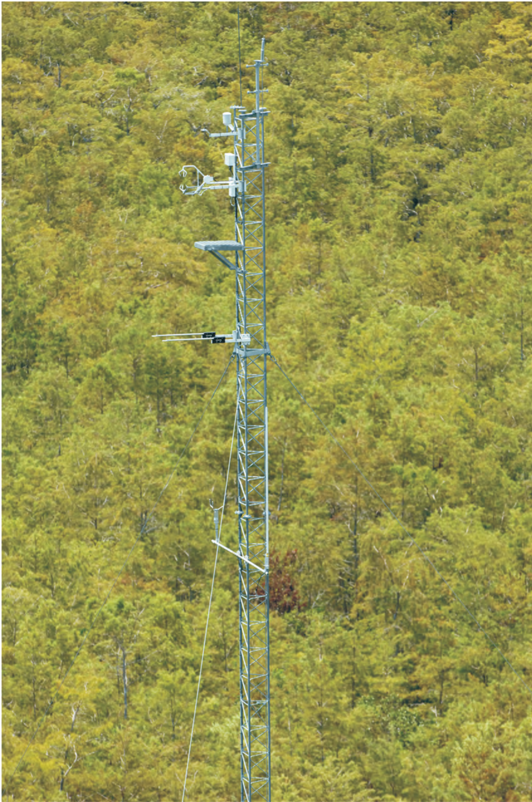
Figure 3. Photographs of the evapotranspiration monitoring stations. Photograph by Patrick Lynch, South Florida Water Management District.—Continued
