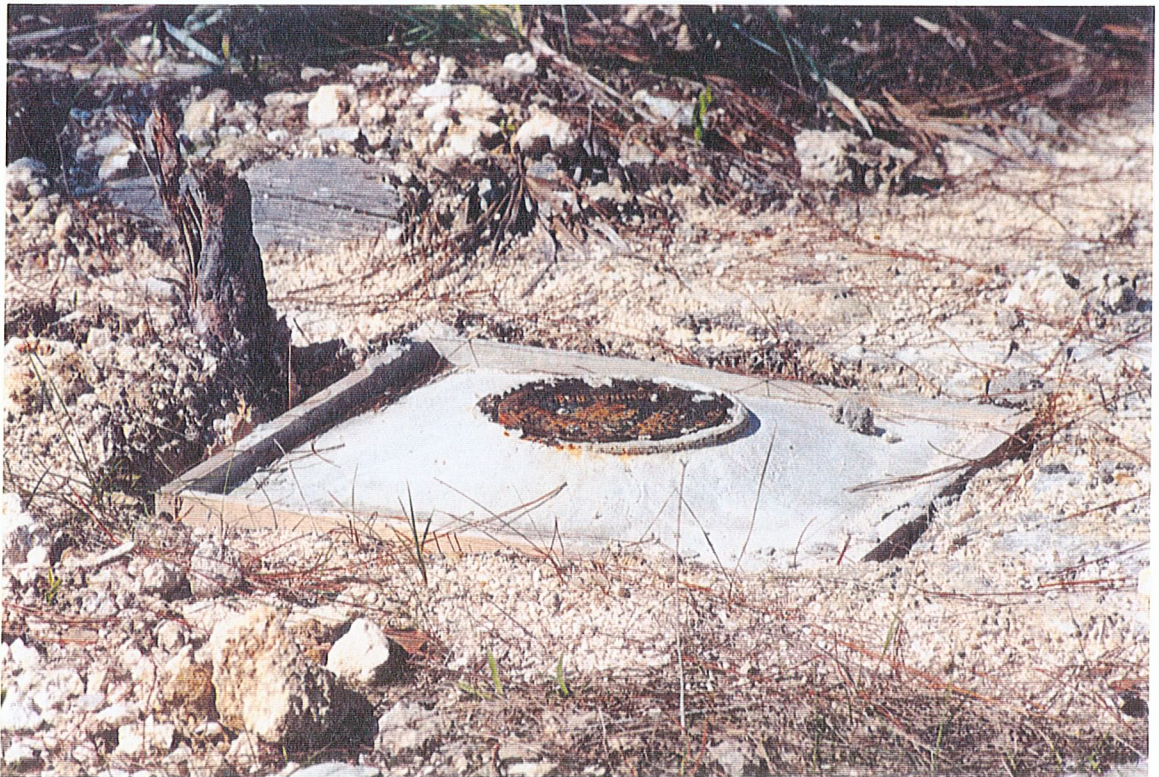
Site 2: Well Installation and View Looking West
