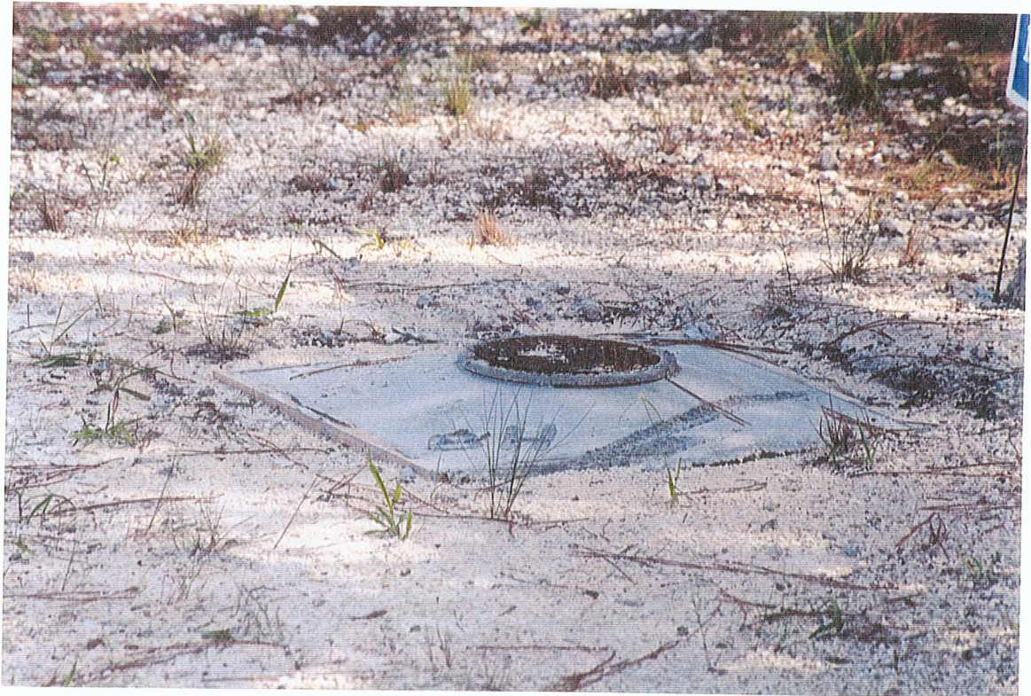
Site 5. Well Installation and View Looking North.
