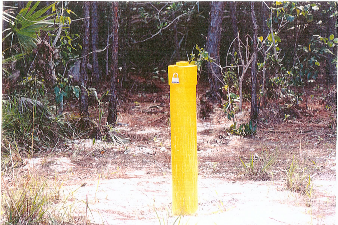
Site 6. Well Installation and View Looking East.
