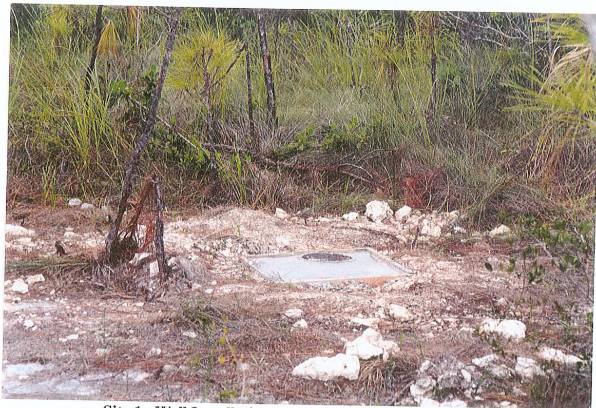
Site 1. Well Installation and View Looking West
