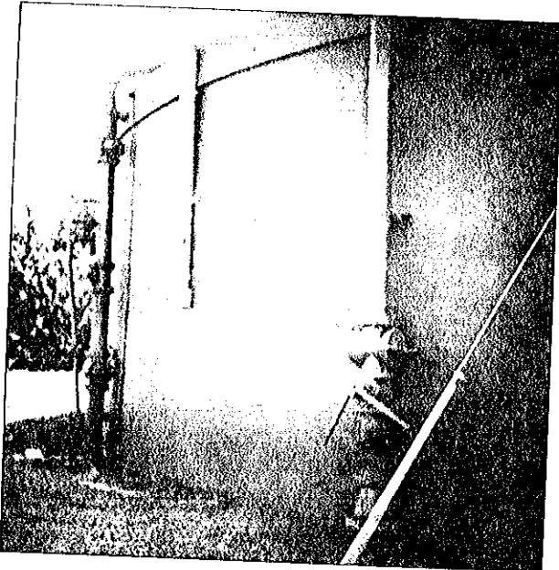
MARCO SHORES GOLF COURSE EFFLUENT TANK WITH RAW WATER LEFT & EFFLUENT WATER LINE RIGHT
