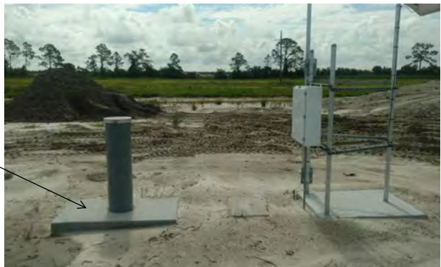
C44B4B Well Site (Looking East)
