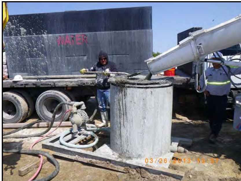
FIGURE 5: 24-INCH SURFACE CASING GROUTING
