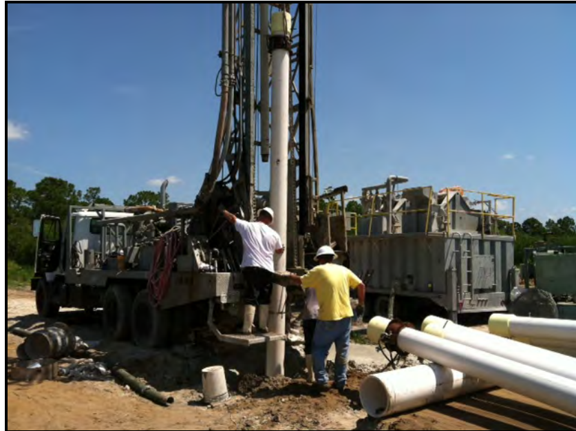
FIGURE 8: PRODUCTION CASING INSTALLATION
