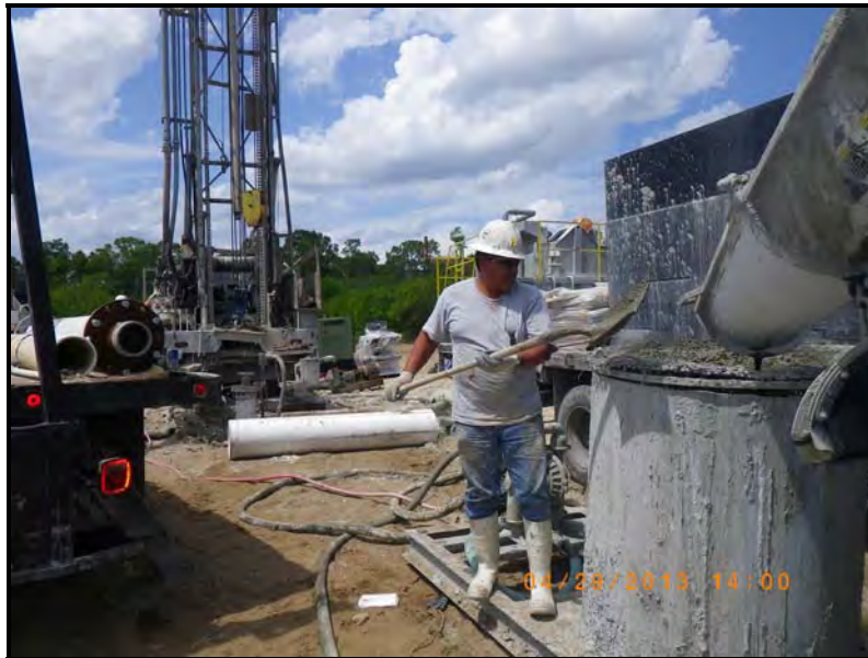
FIGURE 9: PRODUCTION CASING GROUTING
