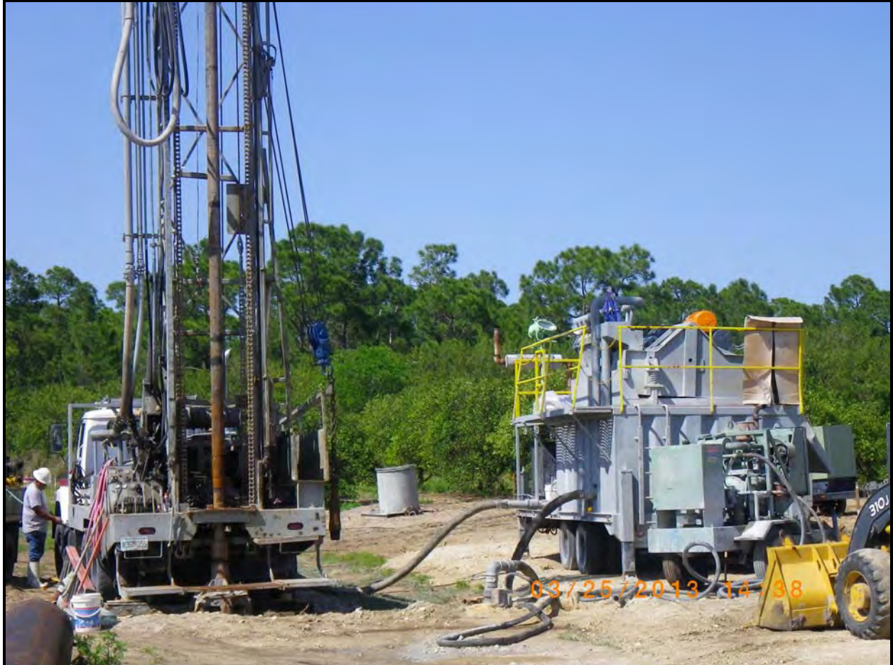
FIGURE 3: WELL DRILLING SET-UP
