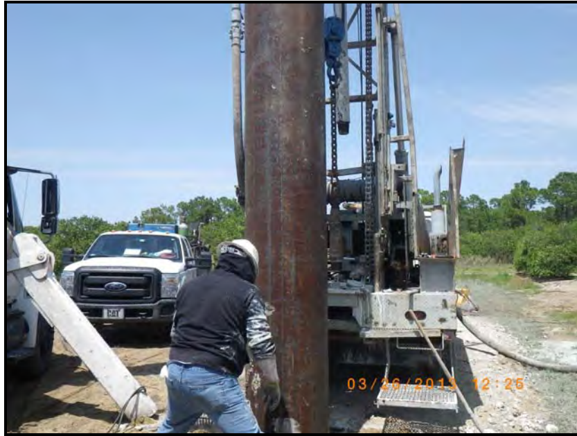
FIGURE 4: 24-INCH SURFACE CASING INSTALLATION
