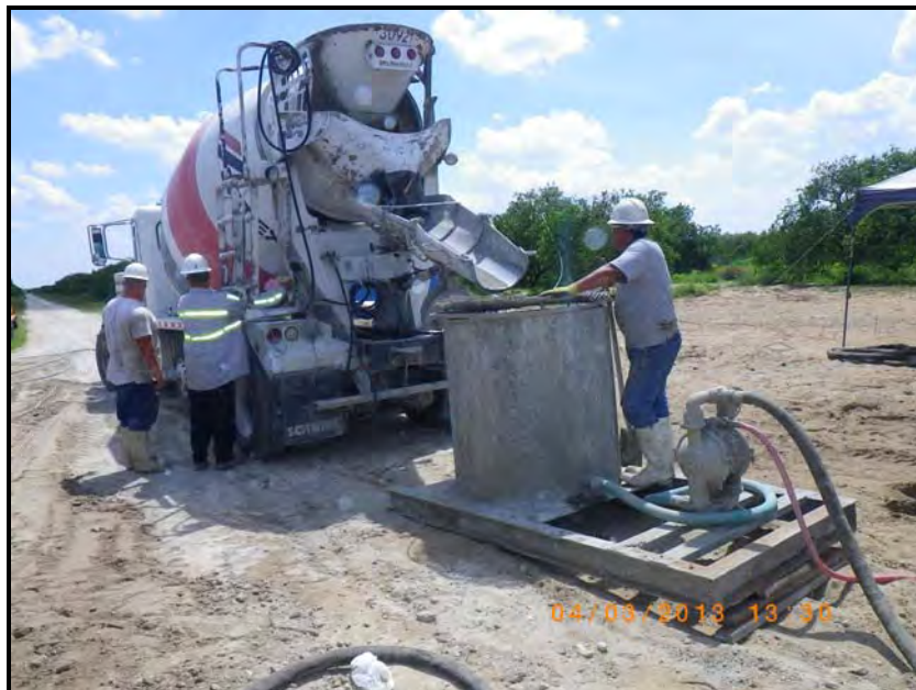
FIGURE 7: INTERMEDIATE CASING GROUTING SET-UP
