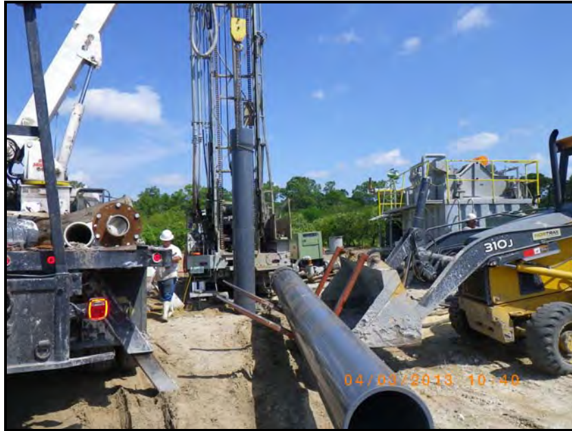
FIGURE 6: 18-INCH INTERMEDIATE CASING INSTALLATION
