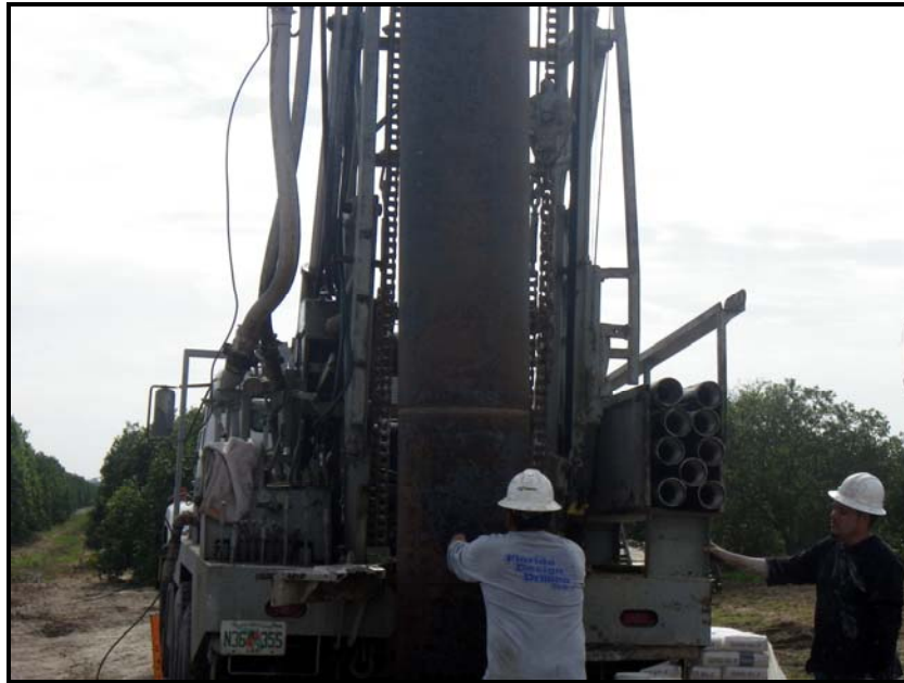
FIGURE 4: 24-INCH SURFACE CASING INSTALLATION
