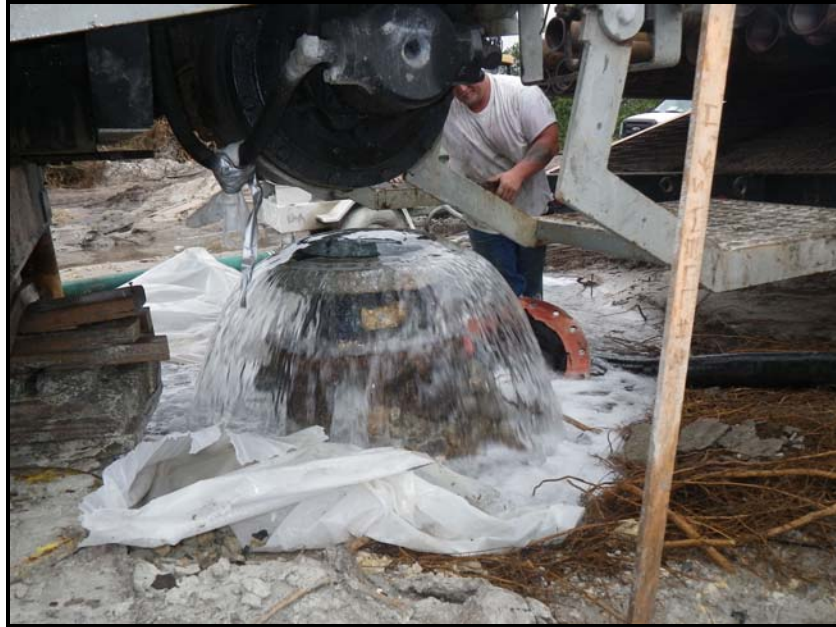
FIGURE 12: FREE FLOW AFTER DEVELOPMENT AIR DEVELOPMENT
