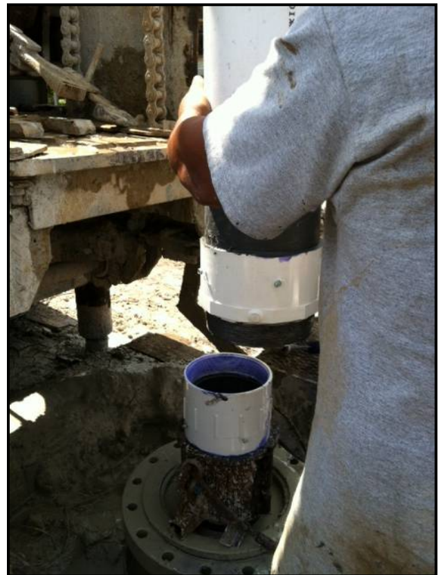
FIGURE 9: TOP 180 FEET CASING-REMOVE
