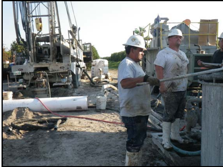
FIGURE 10: PRODUCTION CASING GROUTING
