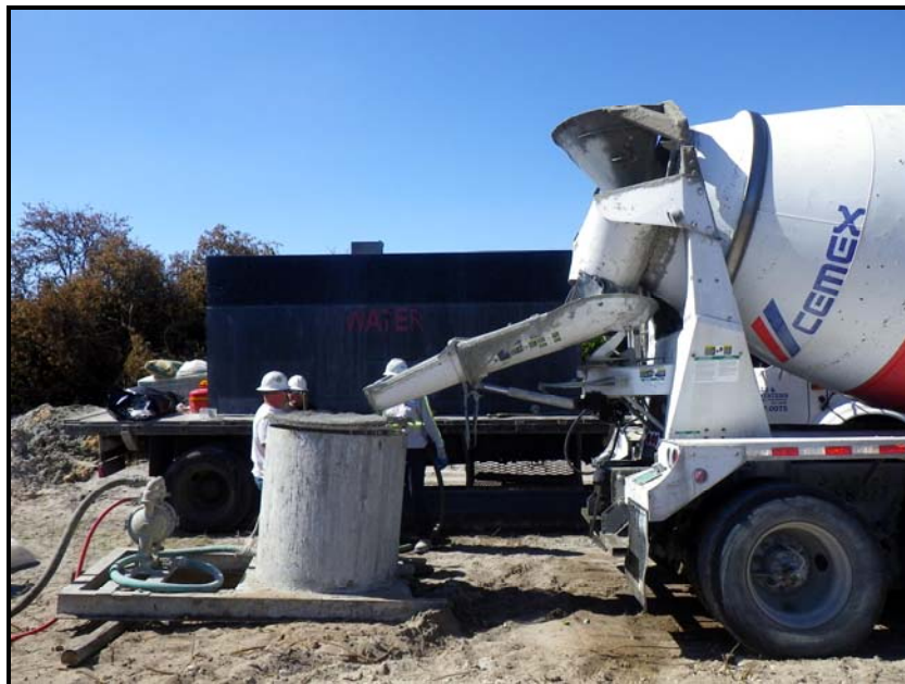
FIGURE 7: INTERMEDIATE CASING GROUTING SET-UP
