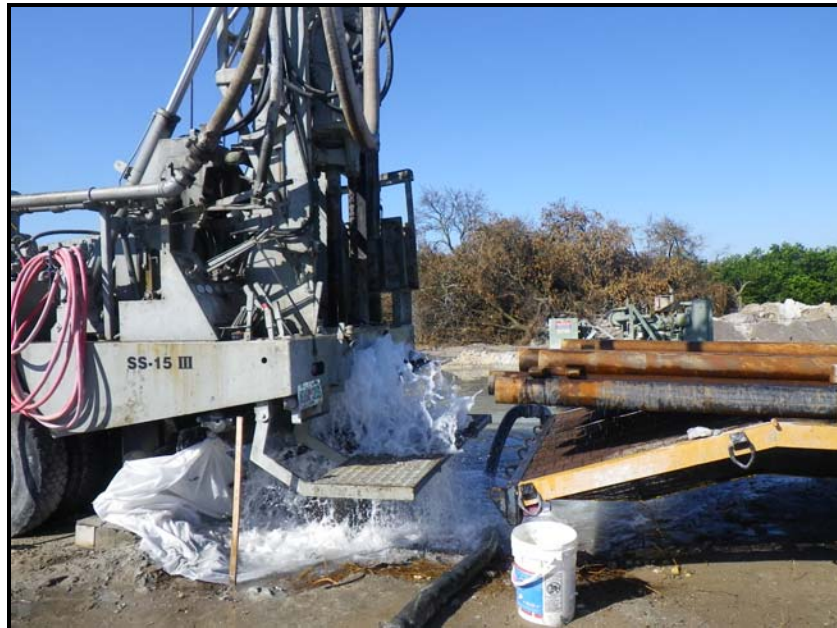
FIGURE 11: AIR DEVELOPMENT ONCE DRILLING MUD THINNED
