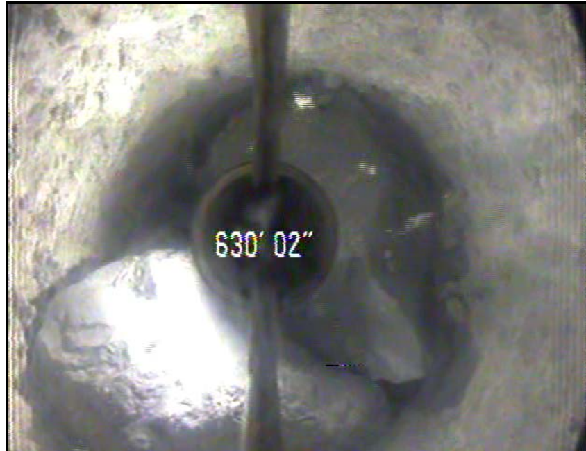
FIGURE 14: OPEN HOLE BLOCKAGE (CEMENT PIECES)
