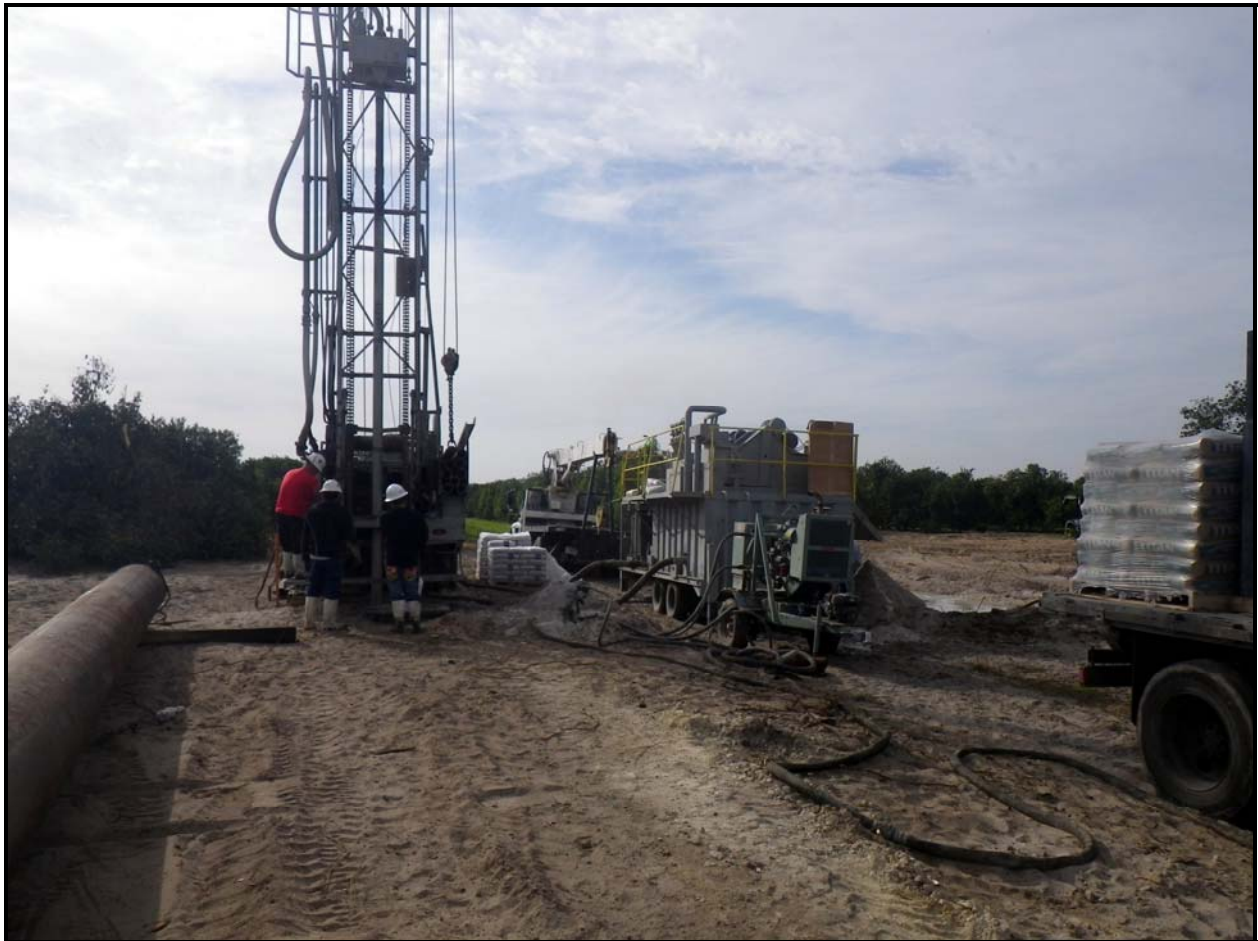
FIGURE 3: WELL DRILLING SET-UP
