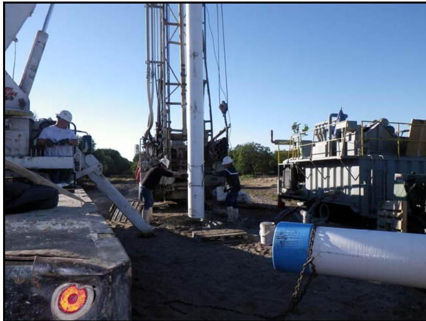
FIGURE 6: 16-INCH INTERMEDIATE CASING INSTALLATION
