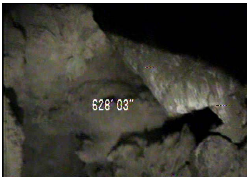
FIGURE 13: VIEW OF CAVITY FROM DOWNHOLE CAMERA
