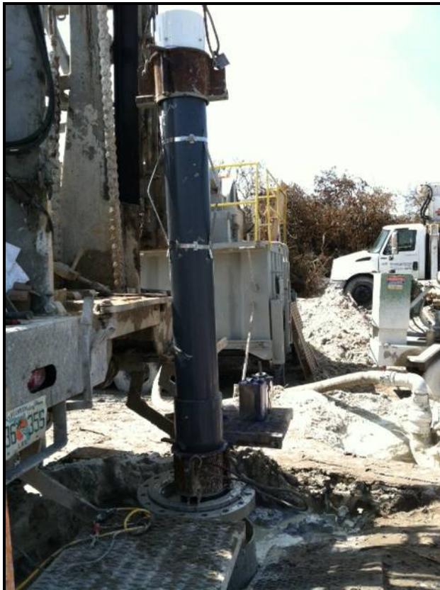
FIGURE 8: PRODUCTION CASING INSTALLATION
