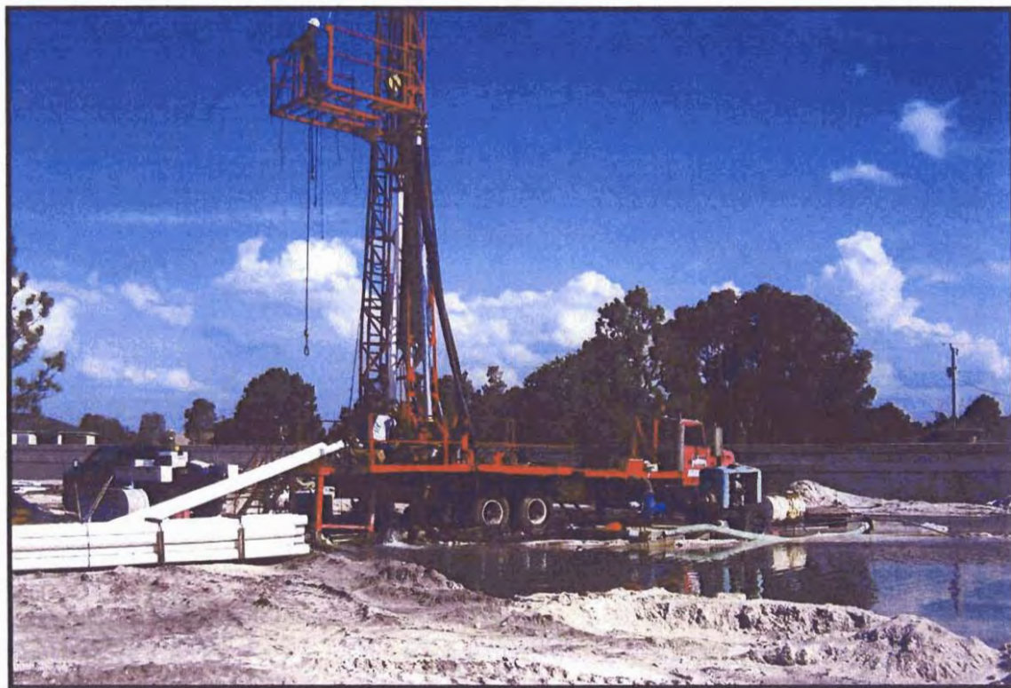
Figure 17 – Installation Set Up of 6-inch PVC Casing
