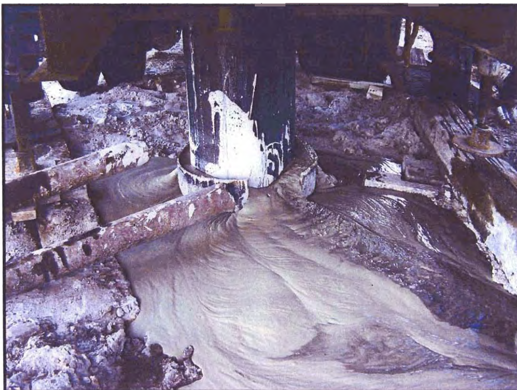
Figure 7 – Grouting of 18-inch Steel Casing
