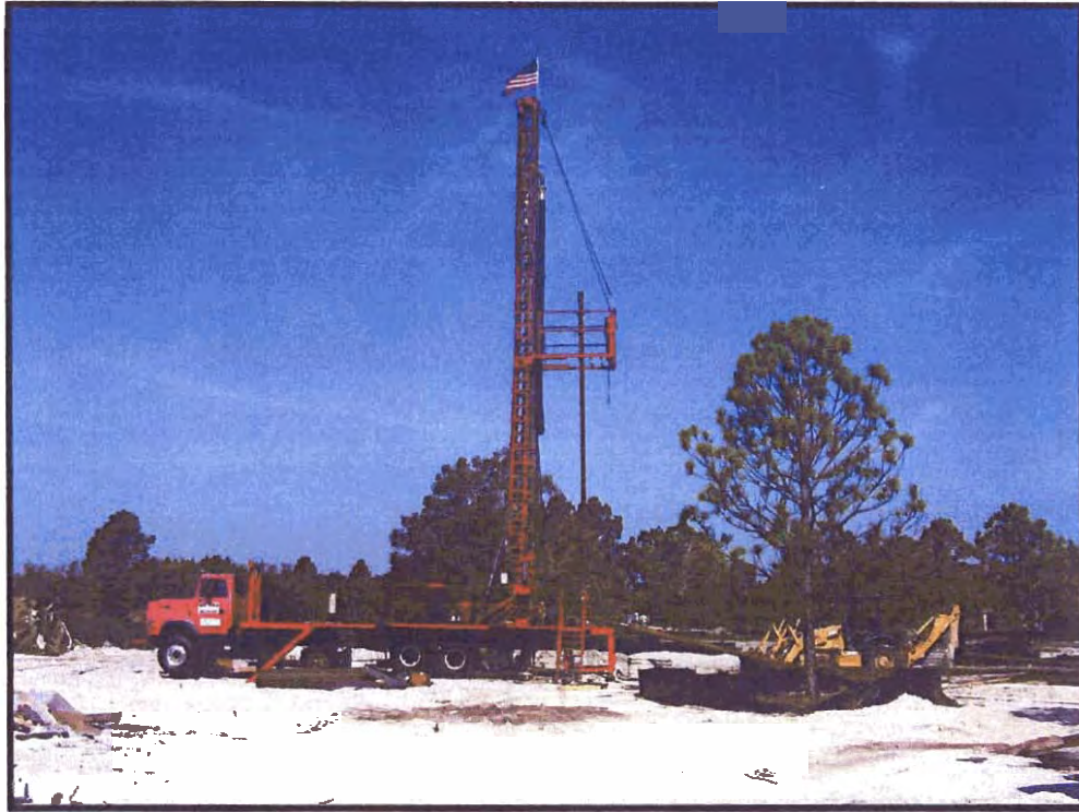
Figure 3 – Gardner Denver 2000 Drill Rig Set Up on ETW-1 (looking west)
