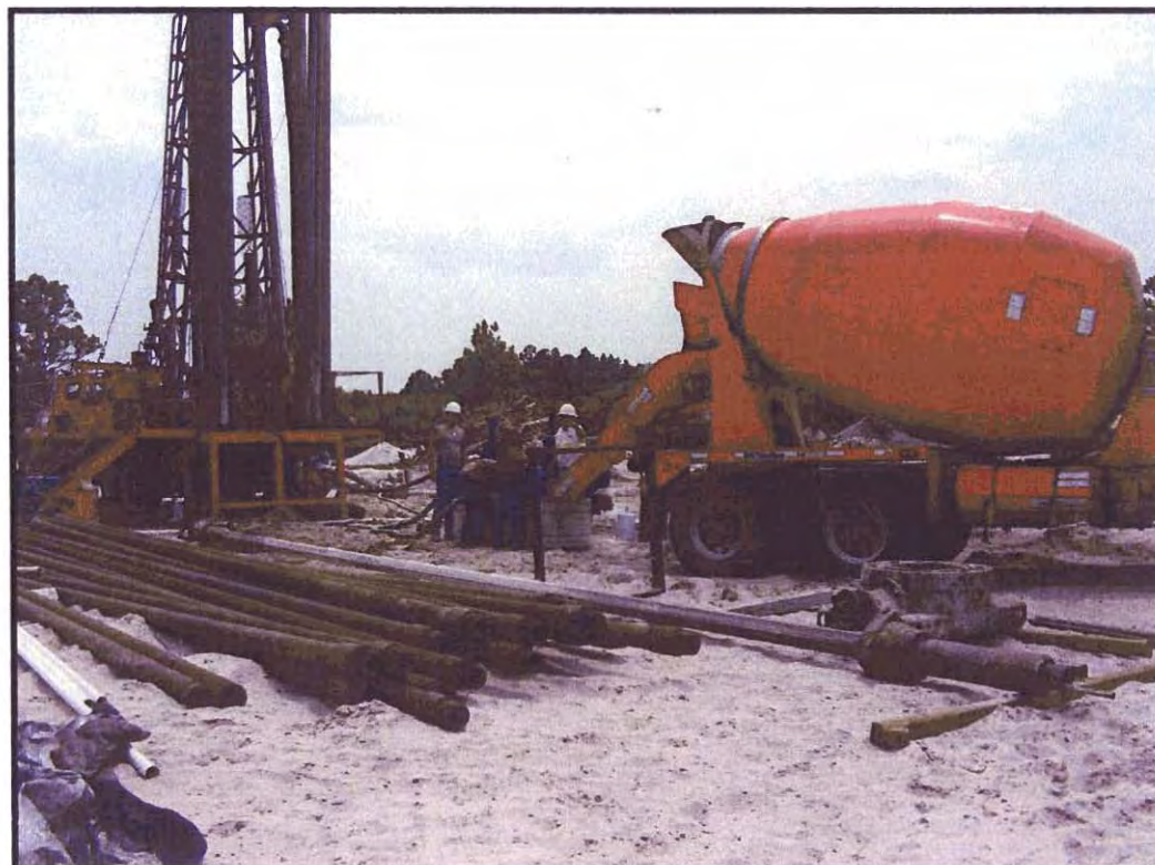
Figure 9 – Grouting of 12-inch Steel Casing
