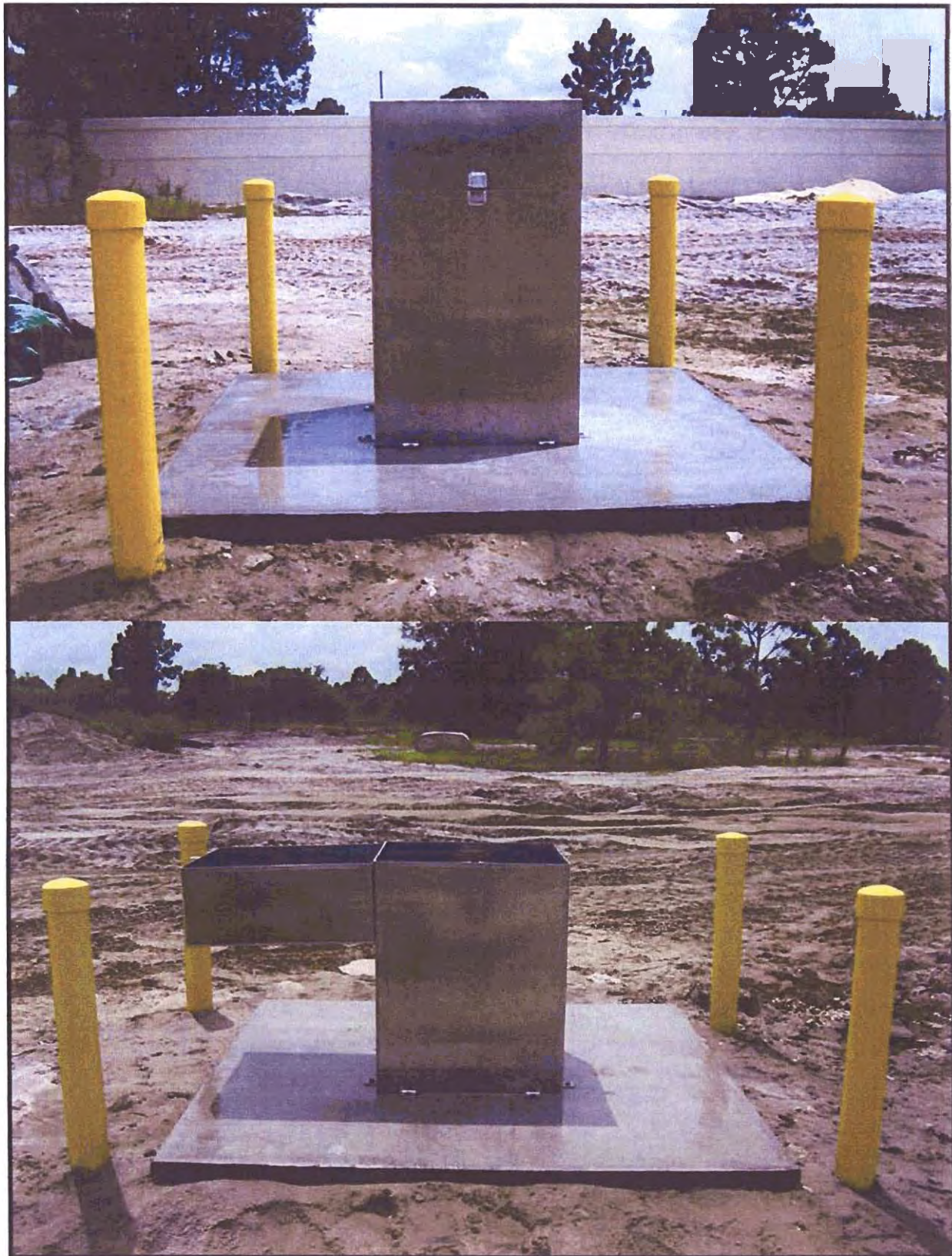
Figure 21 – Wellhead Enclosure and Concrete Slab
