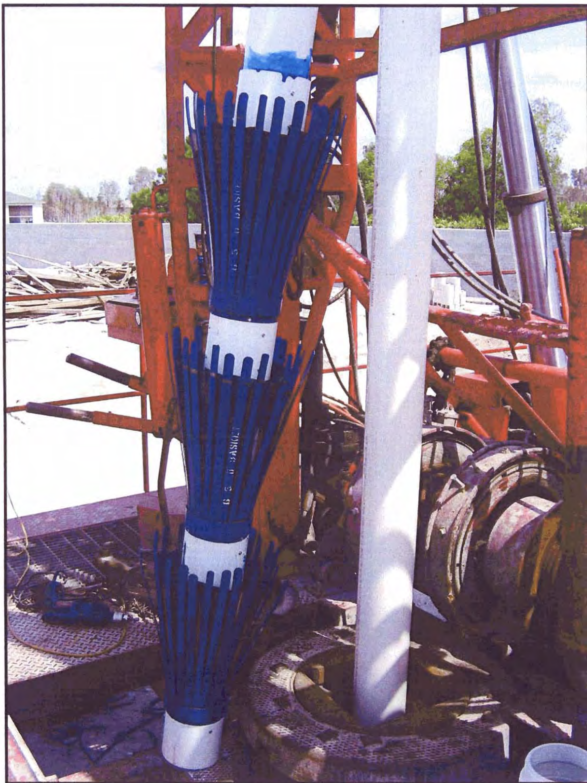
Figure 14 – Cement Baskets Attached to Base of 6-Inch PVC Casing
