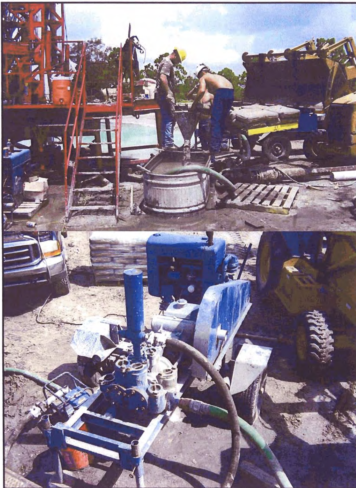
Figure 18 – Grout Mixing and Grout Pump for 6-inch PVC Casing
