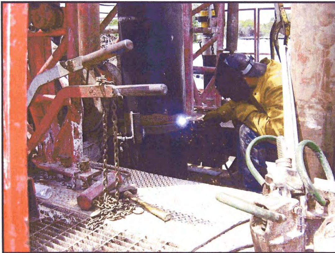
Figure 6 – Welding 18-inch Steel Casing
