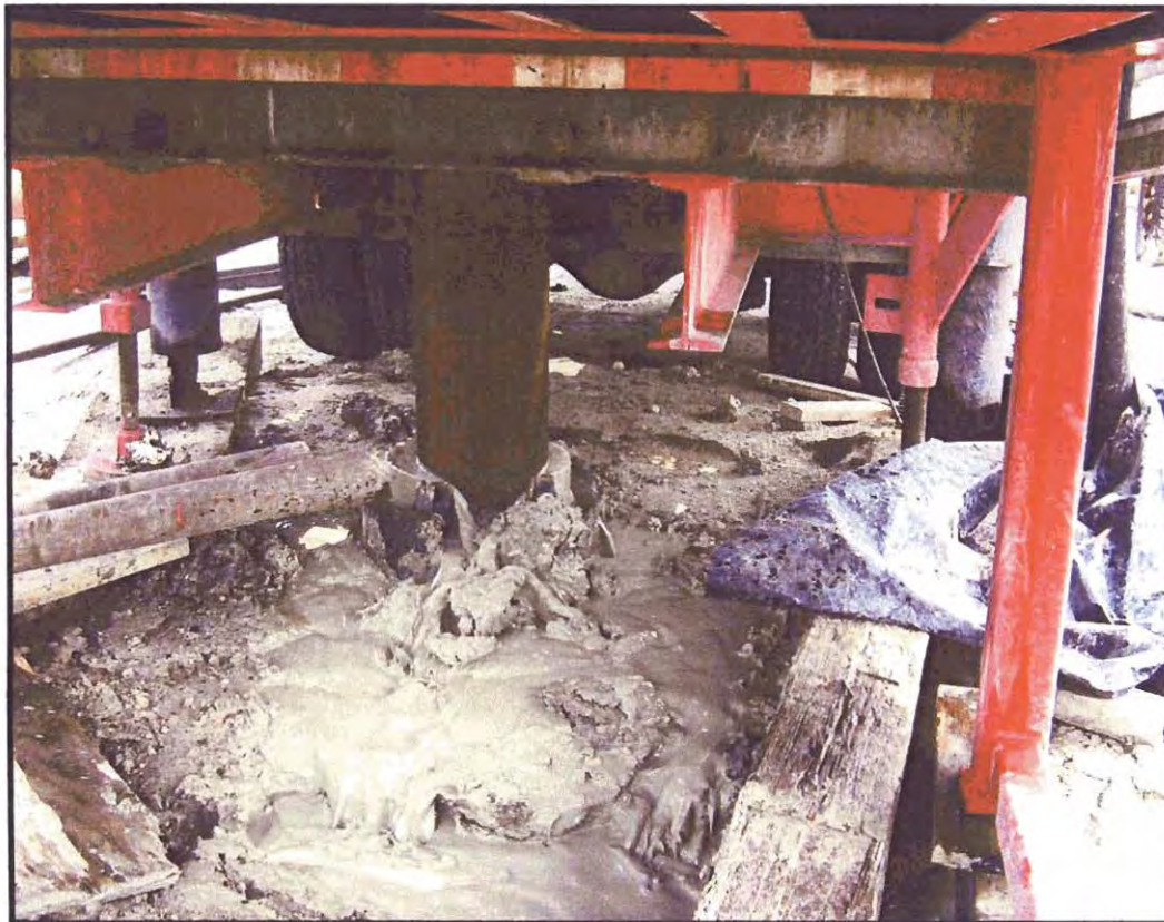
Figure 8 – Circulating Drilling Mud Prior to Grouting of 12-inch Casing
