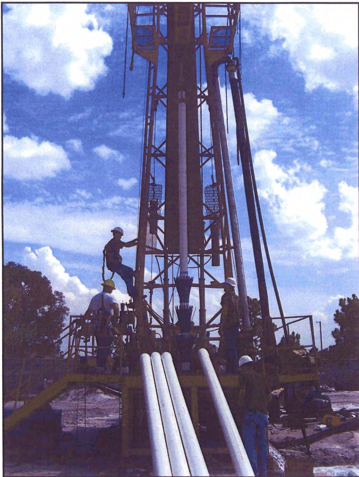
Figure 15 – Installing First Section of 6-inch PVC Casing (note baskets attached)
