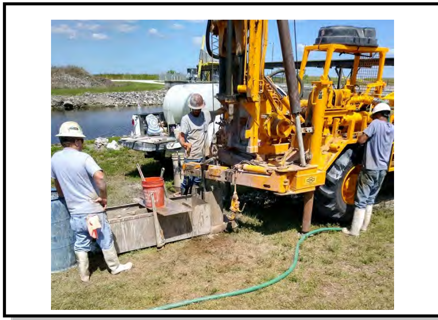
Photo No. 4: B-11 Facing southeast
