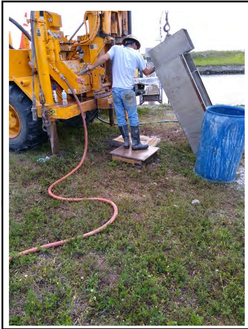
Photo No. 5: B-12 Facing northeast
