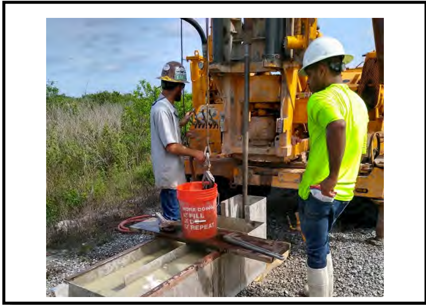
Photo No. 3: B-9 Facing north
