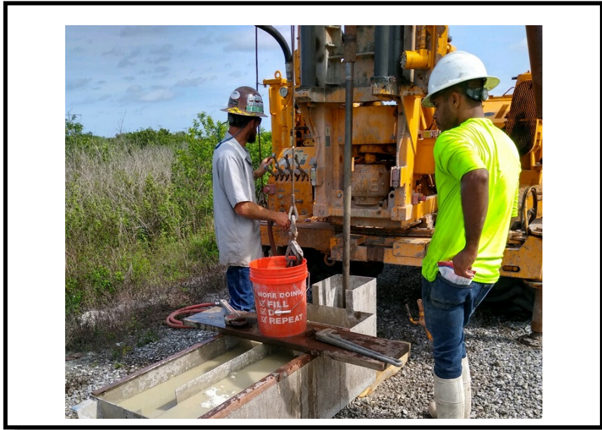
Photo No. 3: B-9 Facing north
