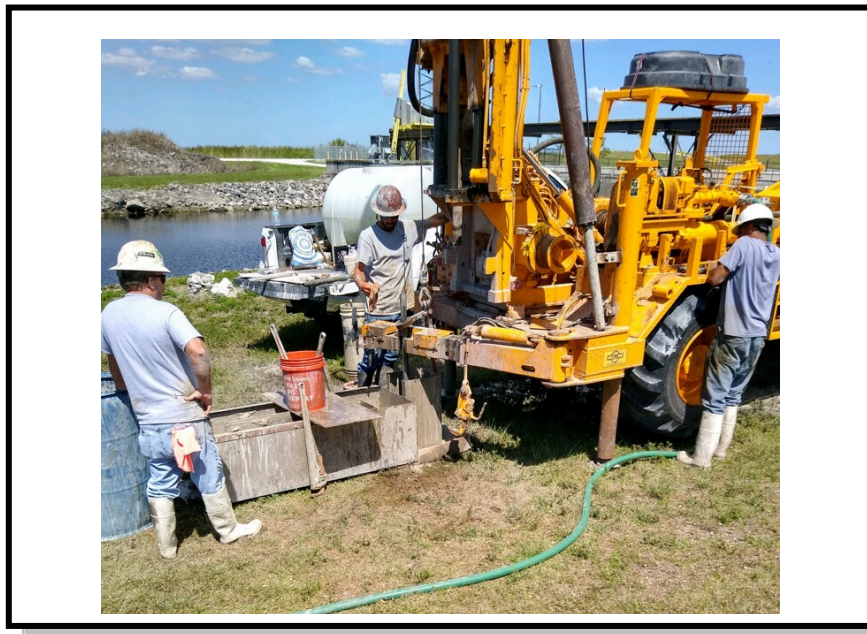
Photo No. 4: B-11 Facing southeast
