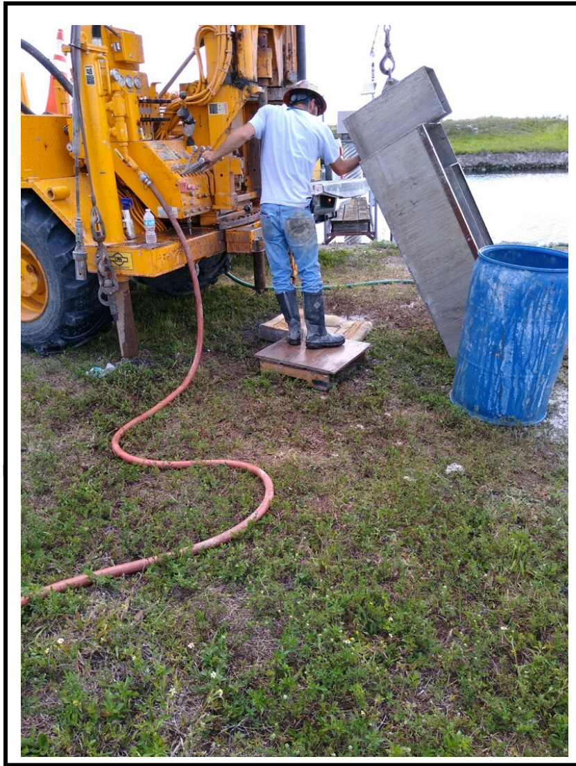
Photo No. 5: B-12 Facing northeast
