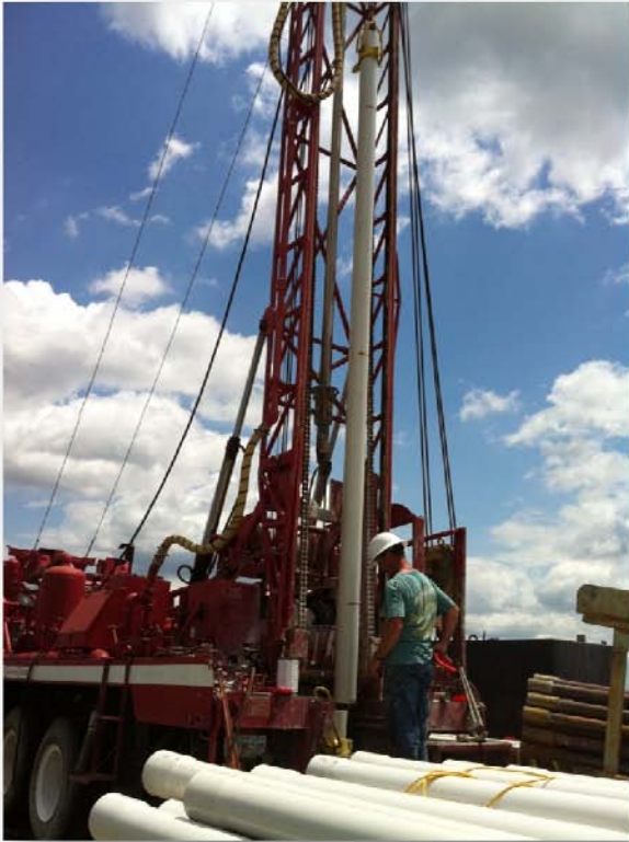
Final casing run for JE-1503.
