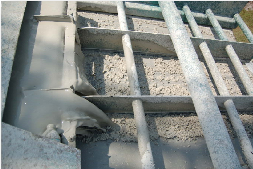
Limestone cuttings removed from drilling mud by orbital shaker.
