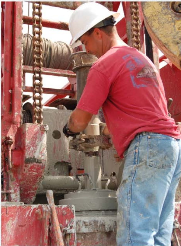
Breaking a connection.
