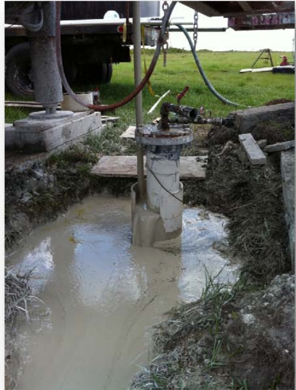
Second stage cement lift on final casing for JE-1503.
