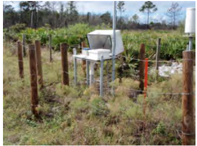
Sensor Well Area:
