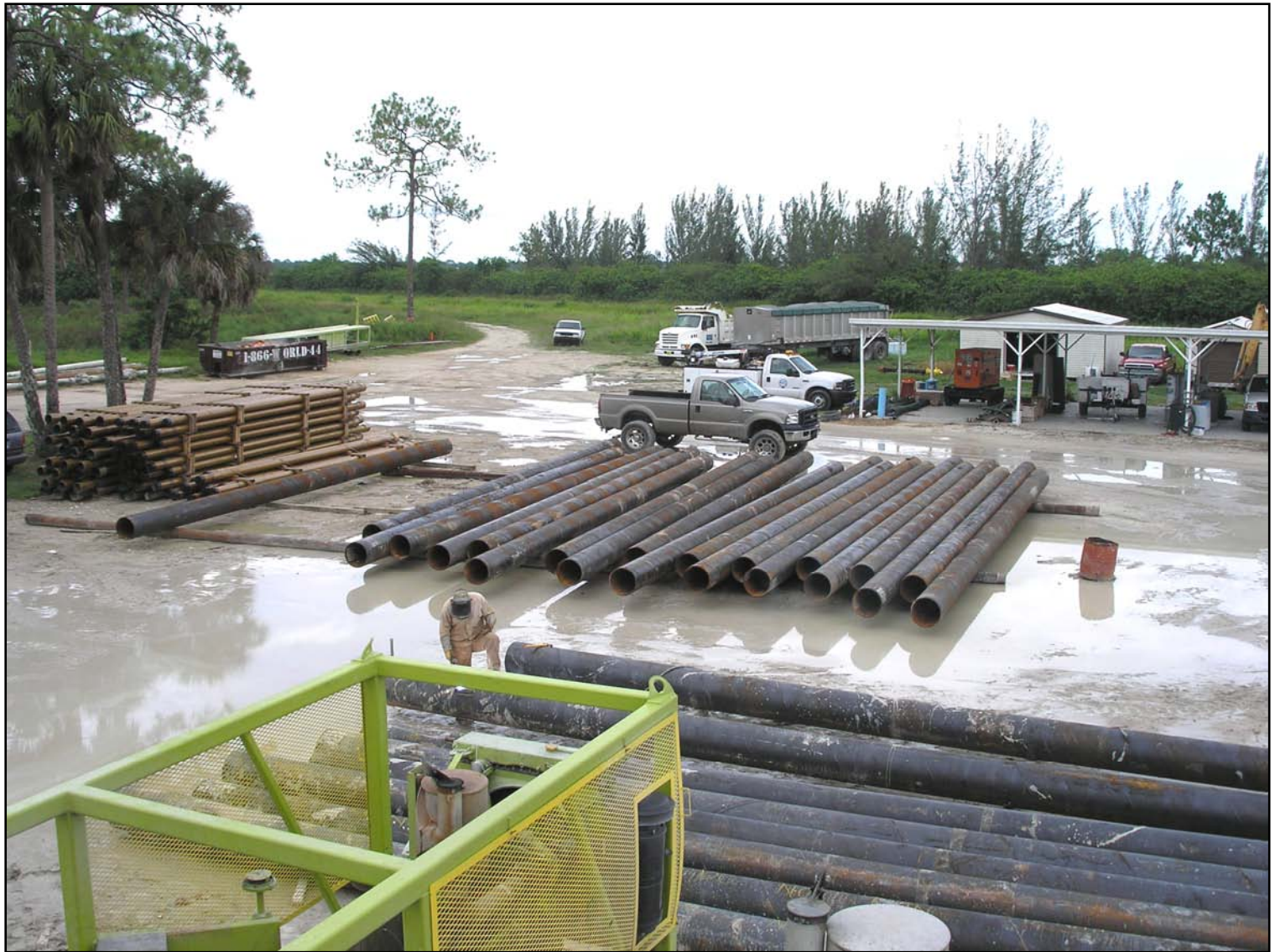
16" INTERMEDIATE CASING
