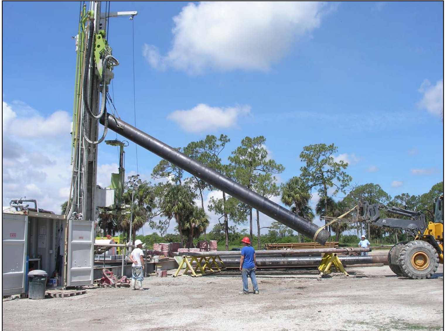
STEEL CASING INSTALLATION
