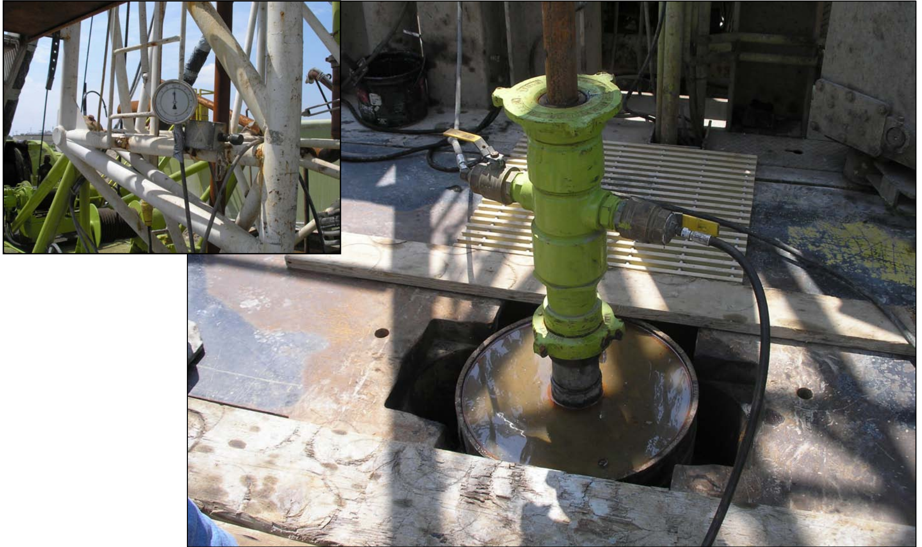
DIW-1 CASING PRESSURE TEST
