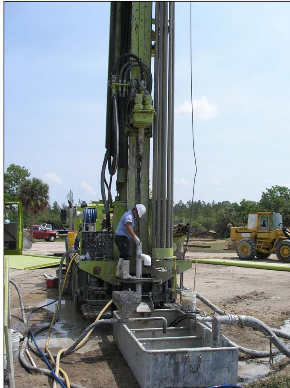
SHALLOW MONITOR WELL DRILLING RIG
