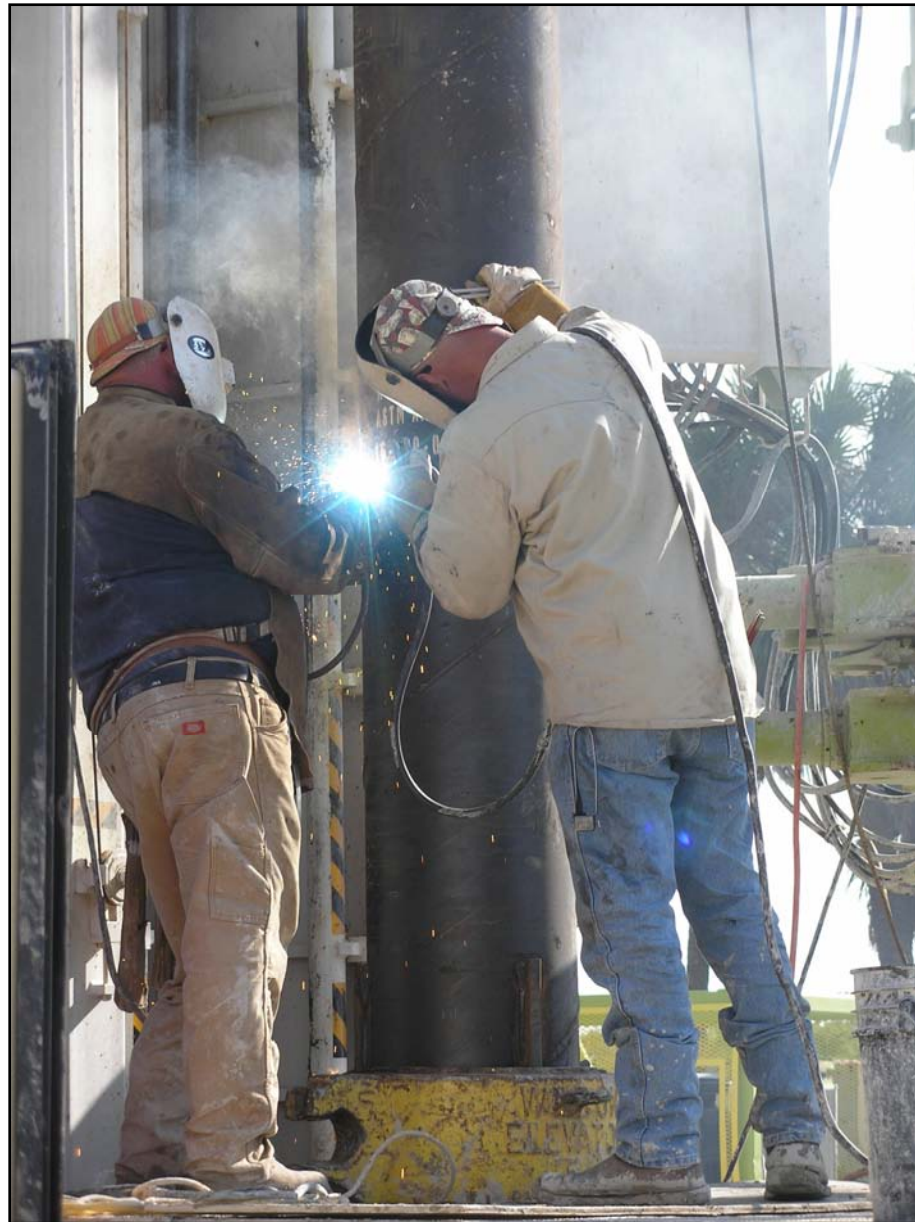
WELDING DURING CASING INSTALLATION
