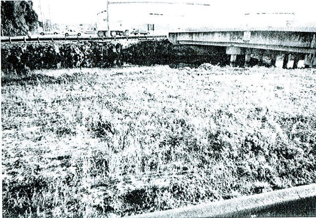
Figure 1. Core Boring CB-5 Location (view to the northeast)
