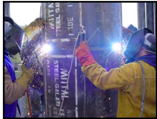
Casing Welding
