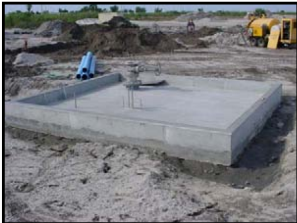
DIW Final Containment Pad
