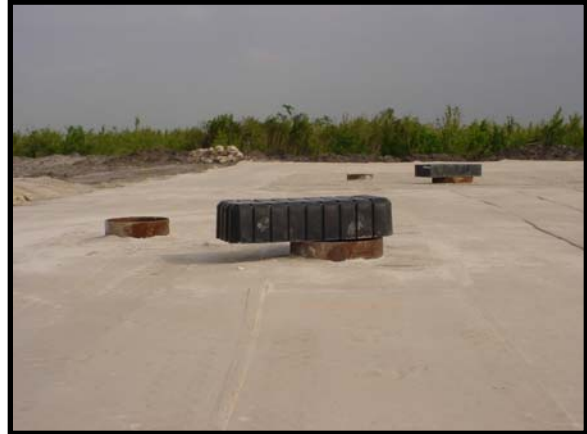
Site Preparation - Pre-Pad Construction
