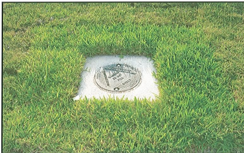
Figure 11 – MW-7 Wellhead Manhole and Pad
