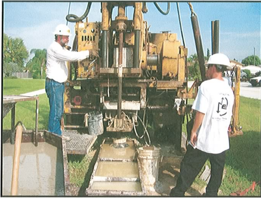
Figure 4 – MW-6 Pilot Hole Drilling
