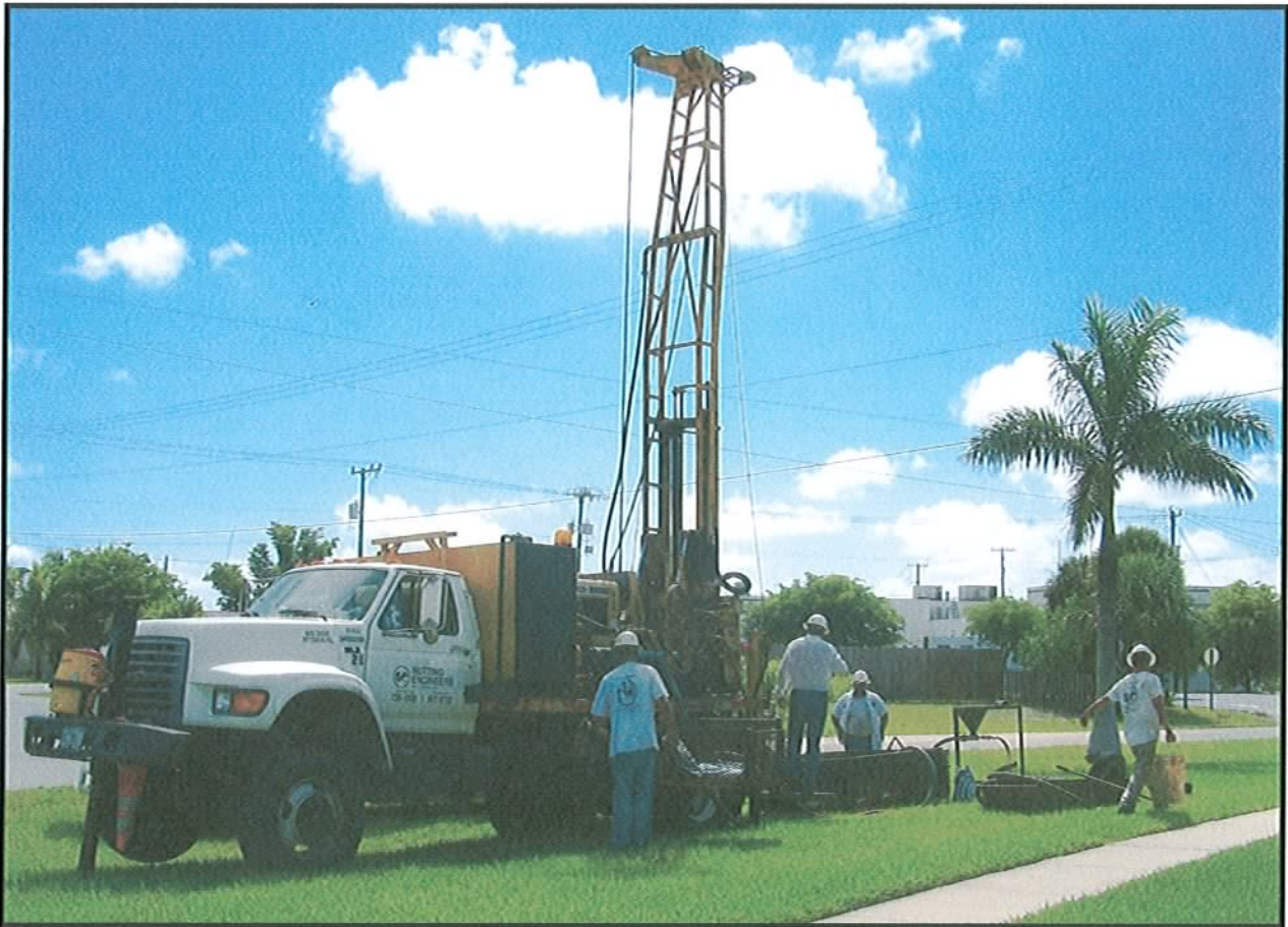
Figure 3 – Mobile B-57 Drill Rig Set Up on MW-6 (looking southeast)
