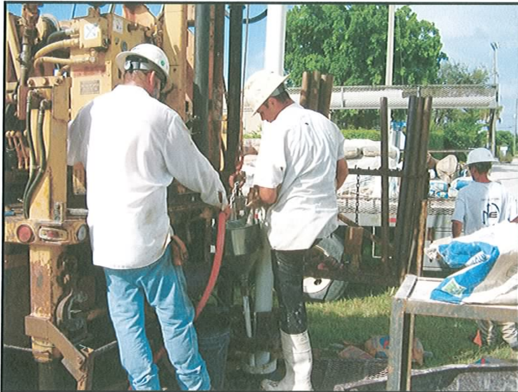
Figure 6 – Adding Filter Pack using Tremie Line
