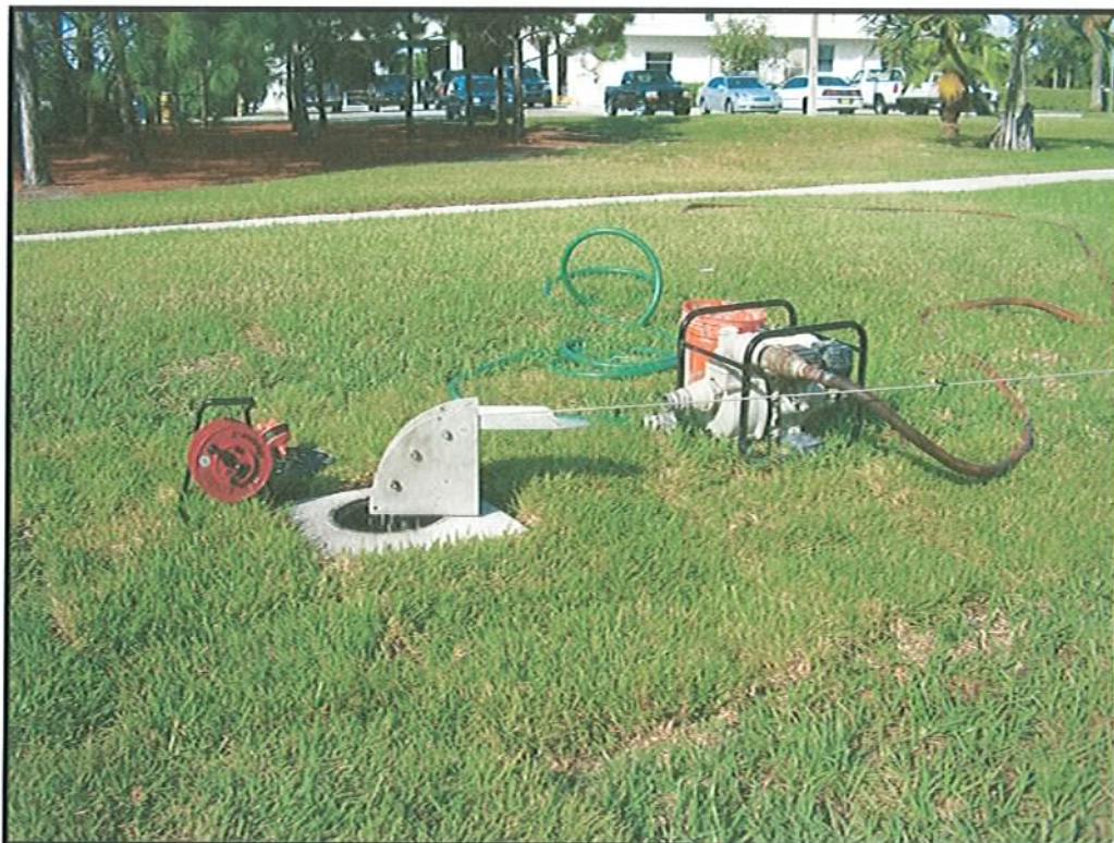
Figure 7 – Completed MW-6 Well Head during Geophysical Logging
