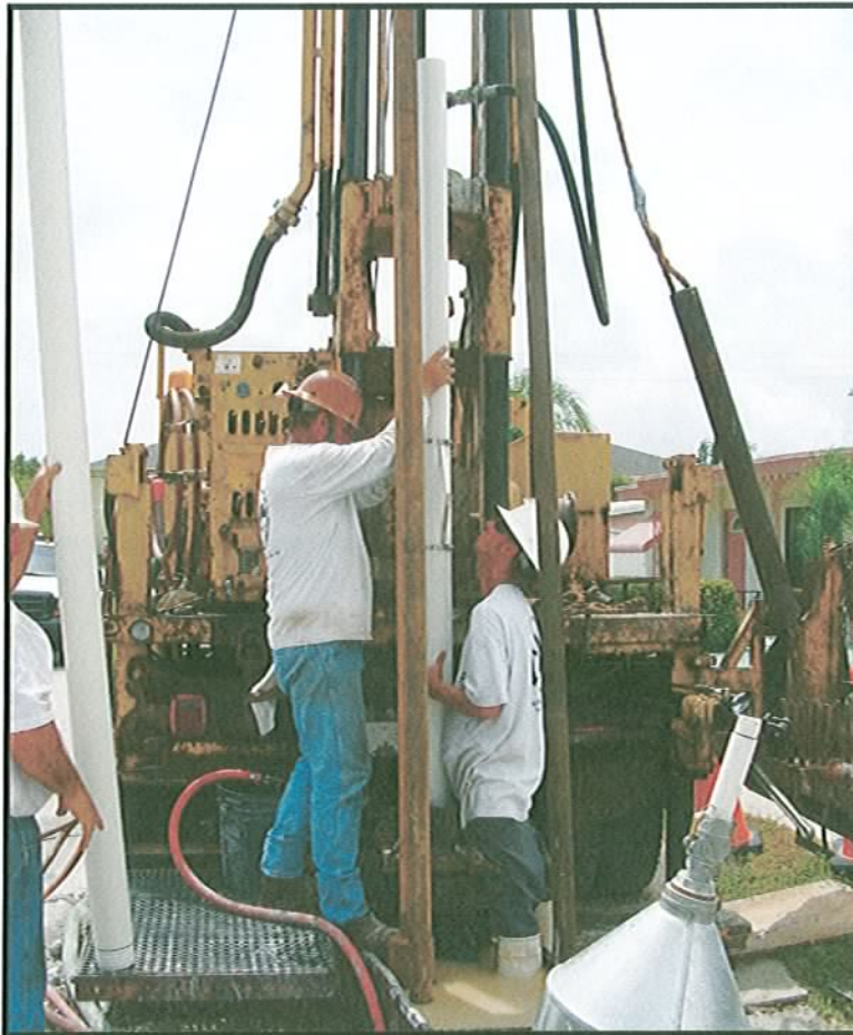
Figure 10 – Installing 4-inch PVC Well Screen and Casing
