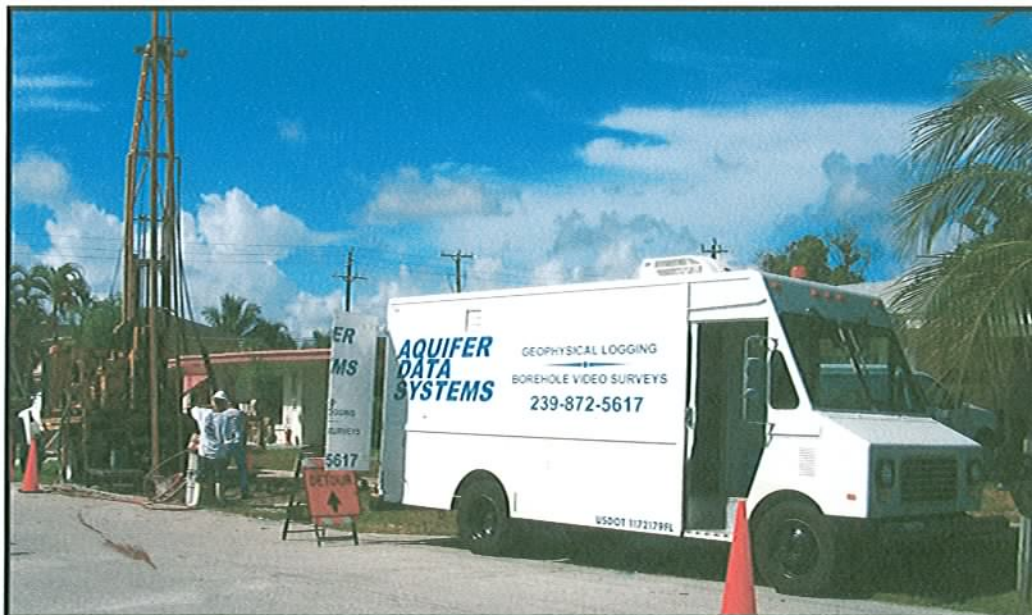
Figure 9 – Geophysical Logging of MW-7 Pilot Hole
