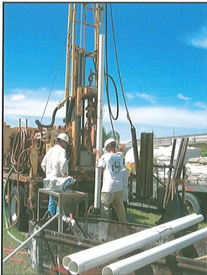
Figure 5 – Installing 4-inch PVC Well Screen and Casing
