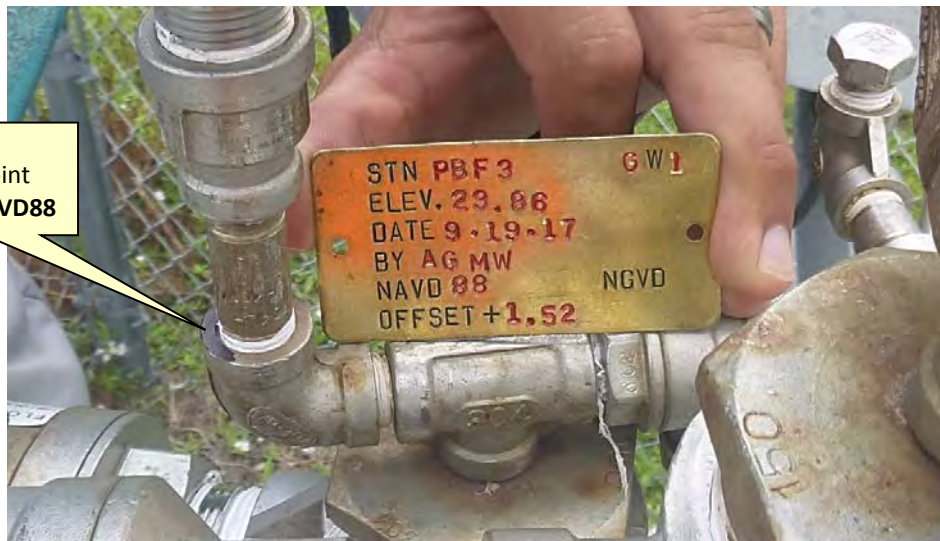
Looking Southerly (oblique not to scale) (19-sep-17)
