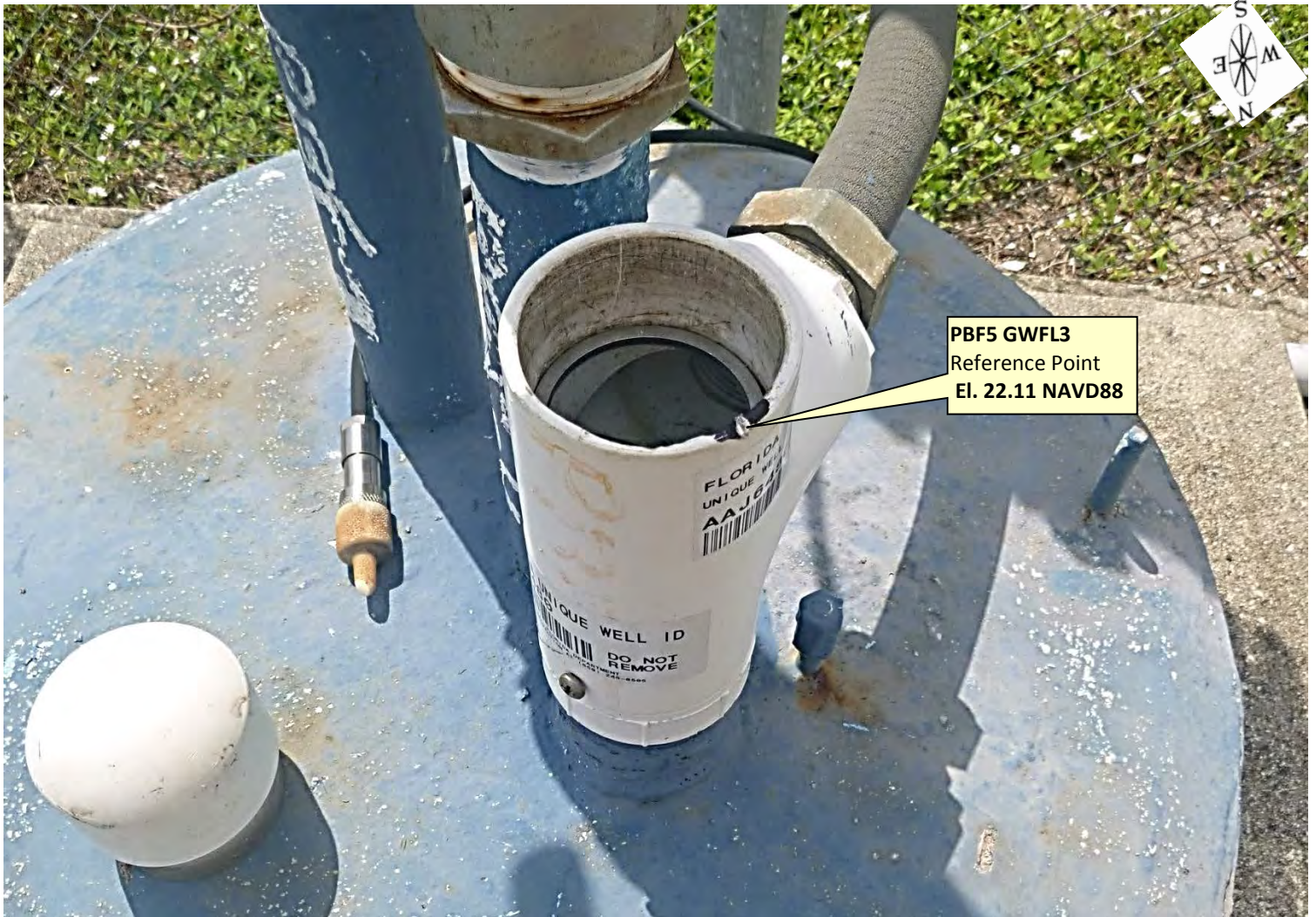
Looking Southerly (oblique not to scale) (19-sep-17)
