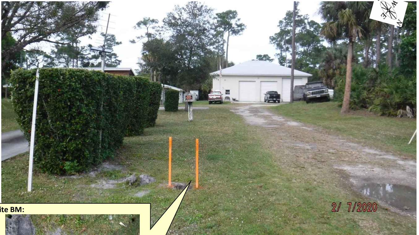
Site Benchmark Overall Photo
