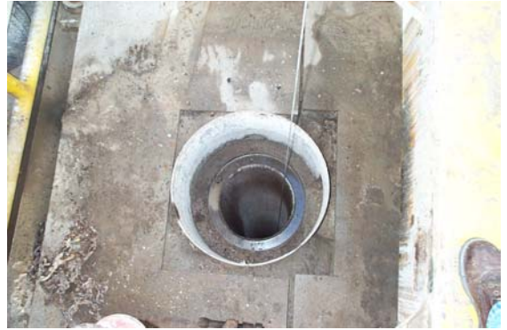
Borehole with steel casing stepped down from 30 to 24 and 18-inch diameter.
