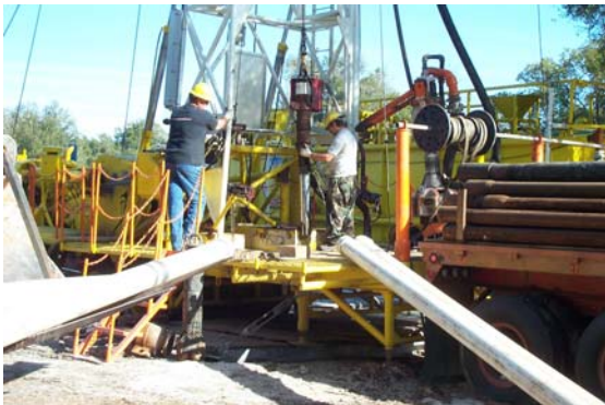
Contractor sets pump for Aquifer Performance Test.
