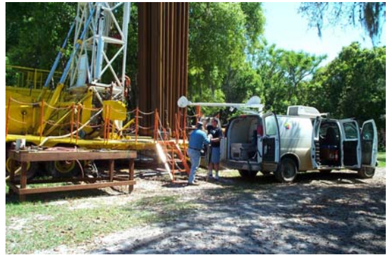
Contractor preps camera for video survey.
