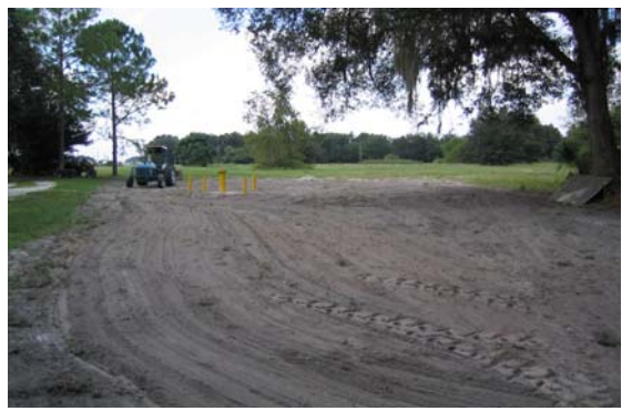
Site restoration after construction, well head and protective bollards in background.
