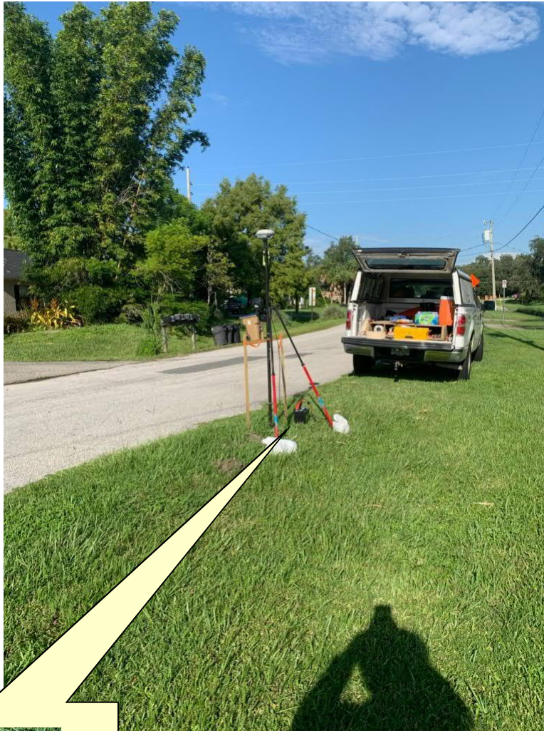
Site Benchmark Overall Photo
