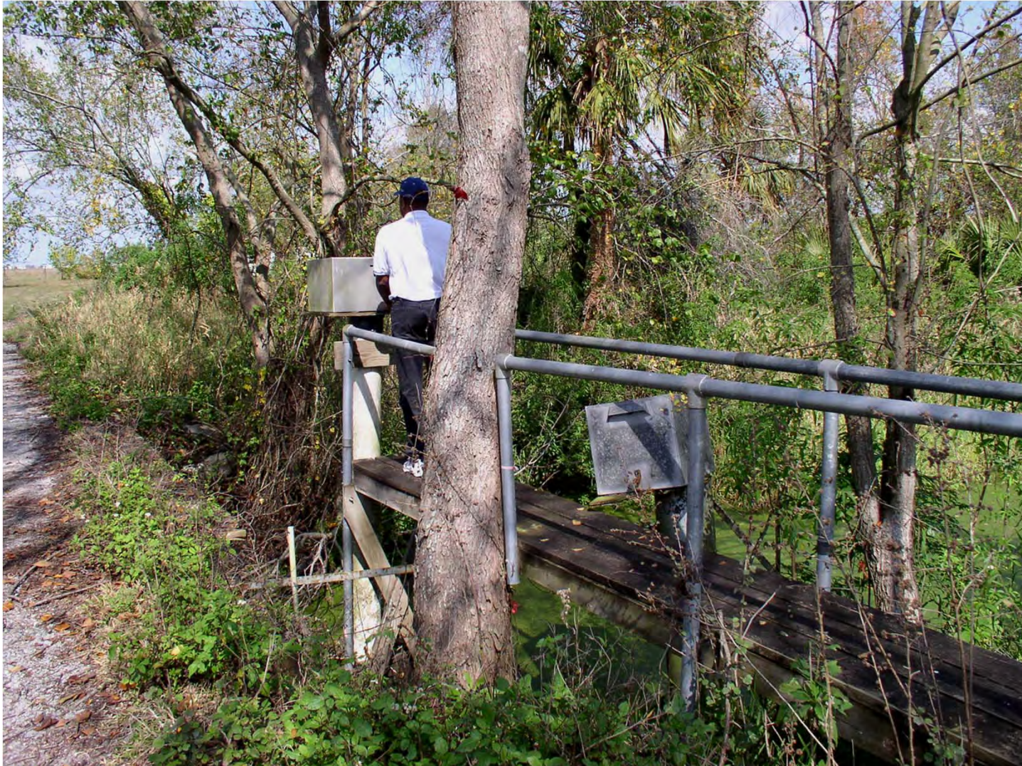
South Florida Water Management District Date of Photo: February 3, 2005 View: Looking Northwesterly at the recorder box
