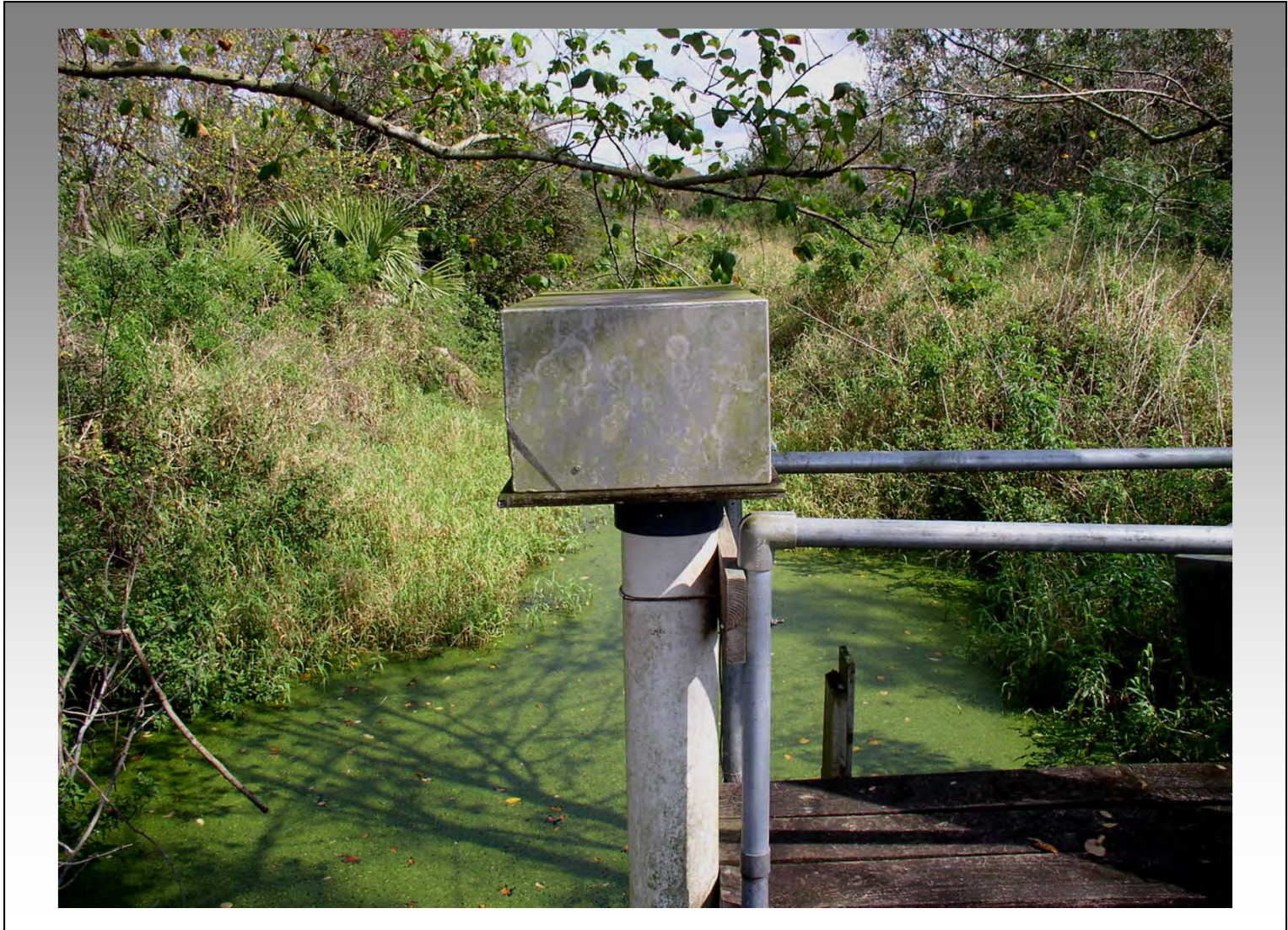
South Florida Water Management District Date of Photo: February 3, 2005 View: Looking northerly at the recorder box
