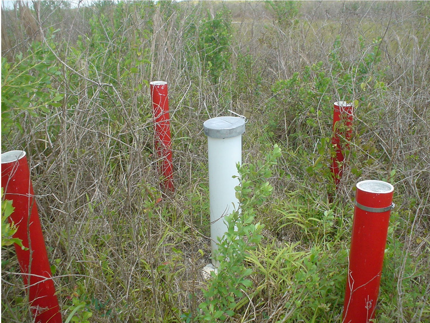
Weidener Surveying & Mapping, P.A. Date of Photo: April 26, 2005 View: Monitoring Well 4A
