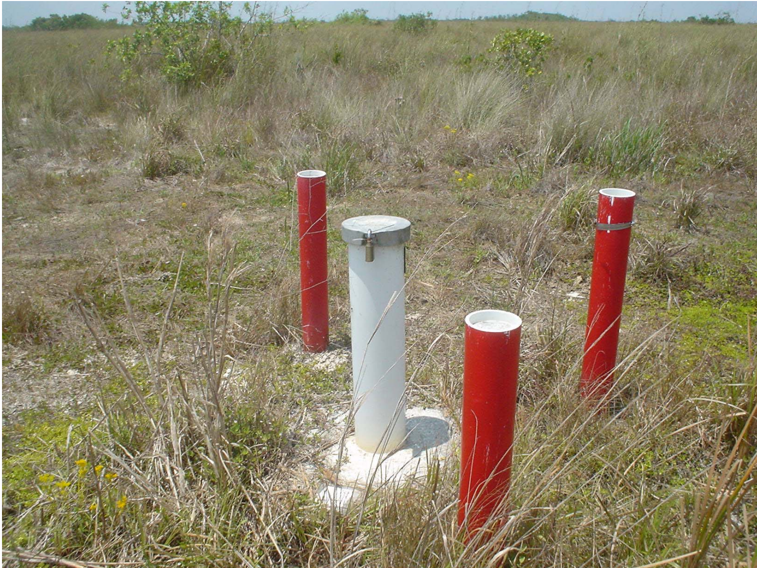
Weidener Surveying & Mapping, P.A. Date of Photo: April 26, 2005 View: Monitoring Well 6A (north)
