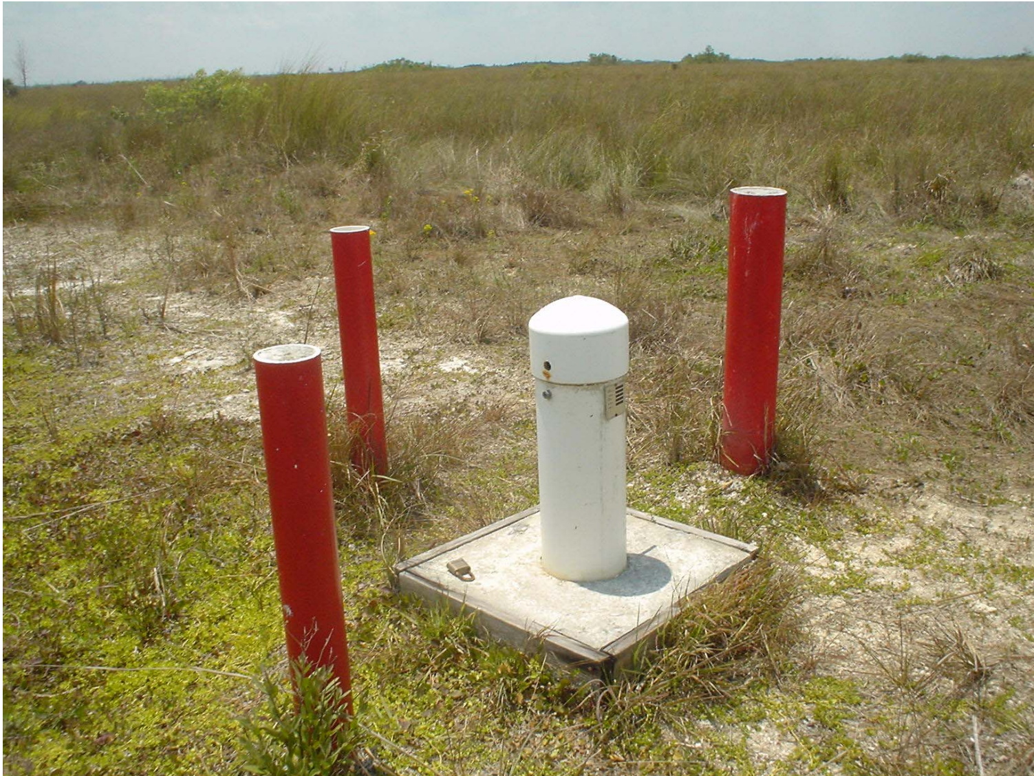
Weidener Surveying & Mapping, P.A. Date of Photo: April 26, 2005 View: Monitoring Well 6B (south)
