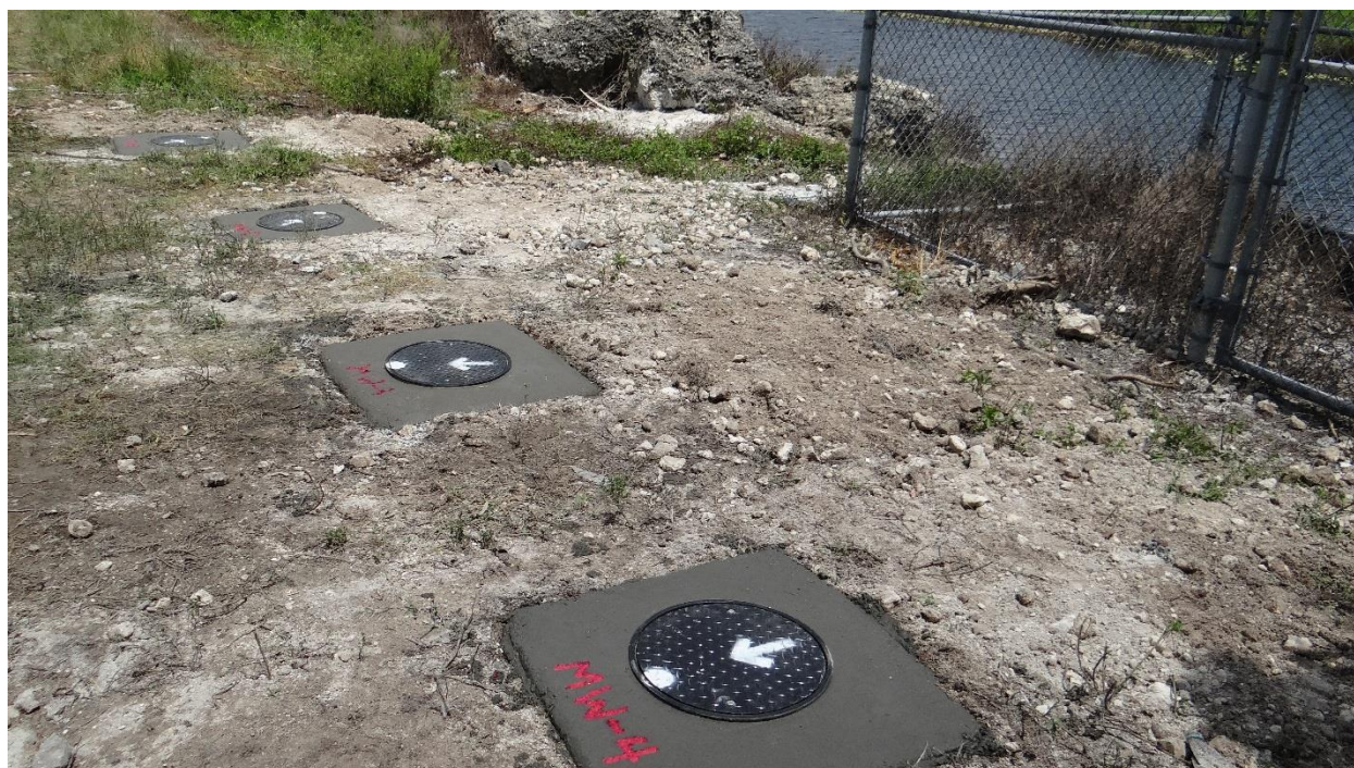
Figure 3. Completed wellheads (photo is looking east-southeast)
