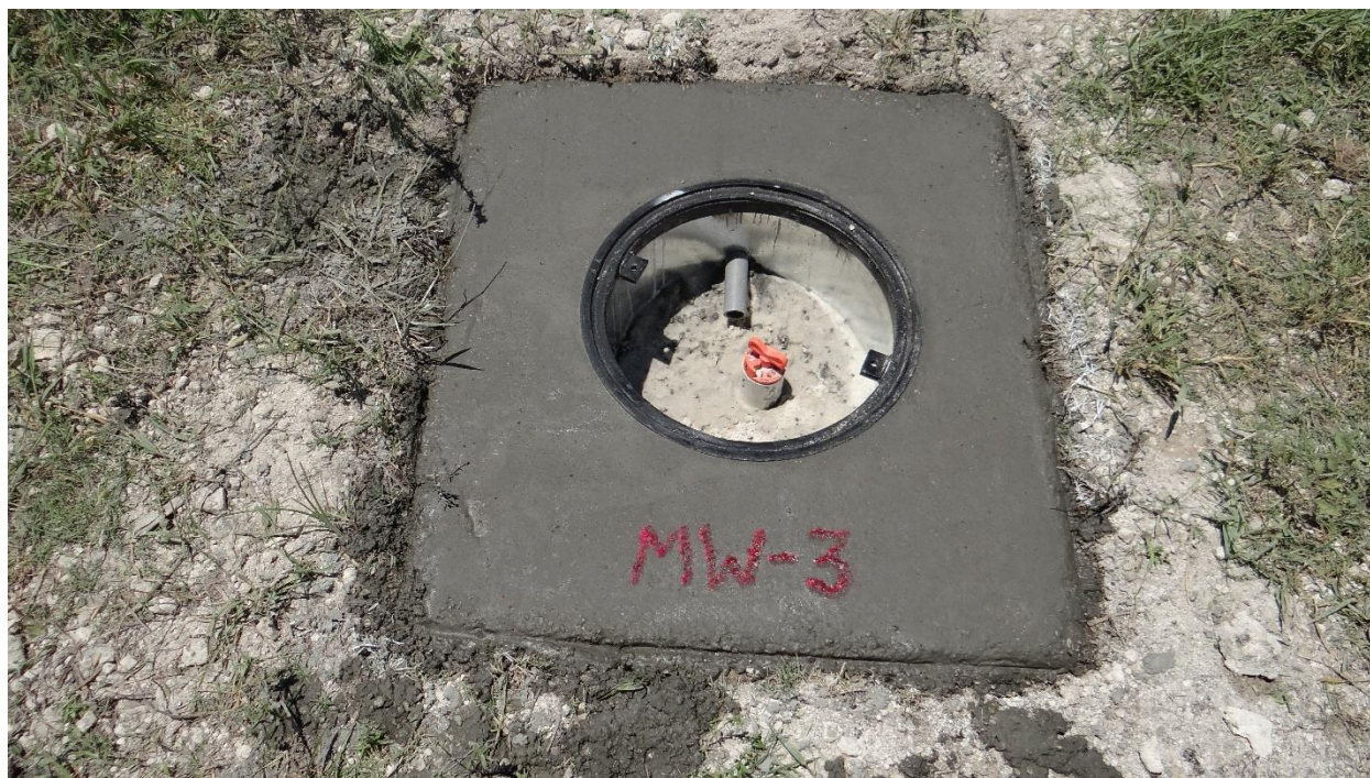
Figure 4. Completed monitoring well
