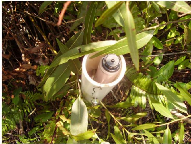
Figure 25: FIU well N4S
