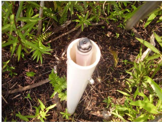
Figure 27: FIU well N5S
