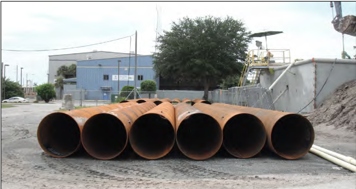
FIGURE 2-10: 40-INCH INTERMEDIATE CASING
