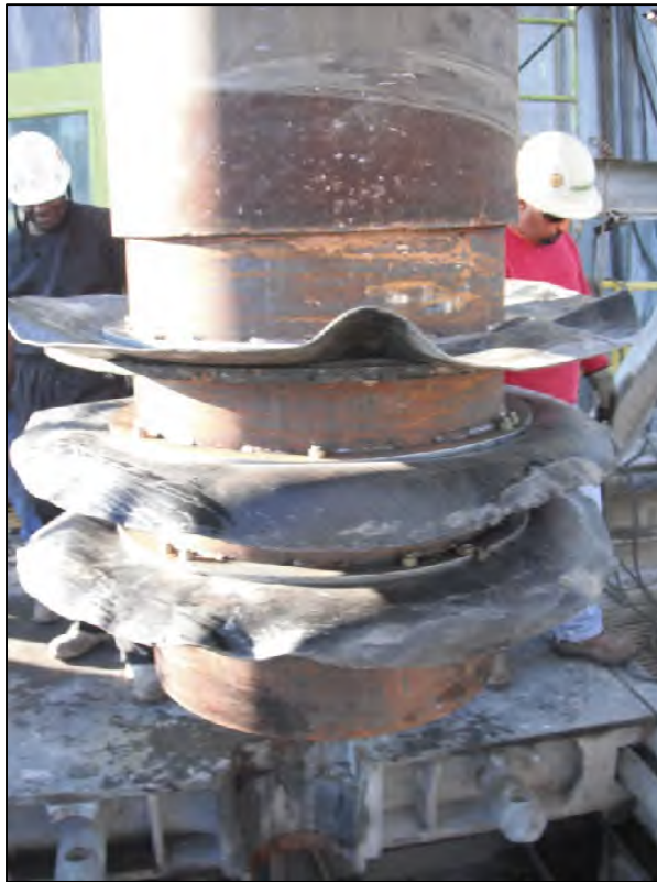
FIGURE 2-21: CEMENTING PACKER FOR INJECTION WELL 28-INCH CASING
