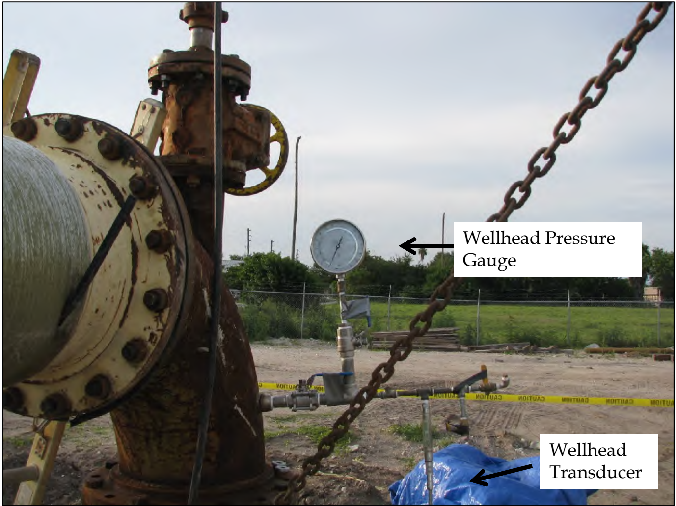
FIGURE 3-34 Pressure Gages at the DIW Wellhead
