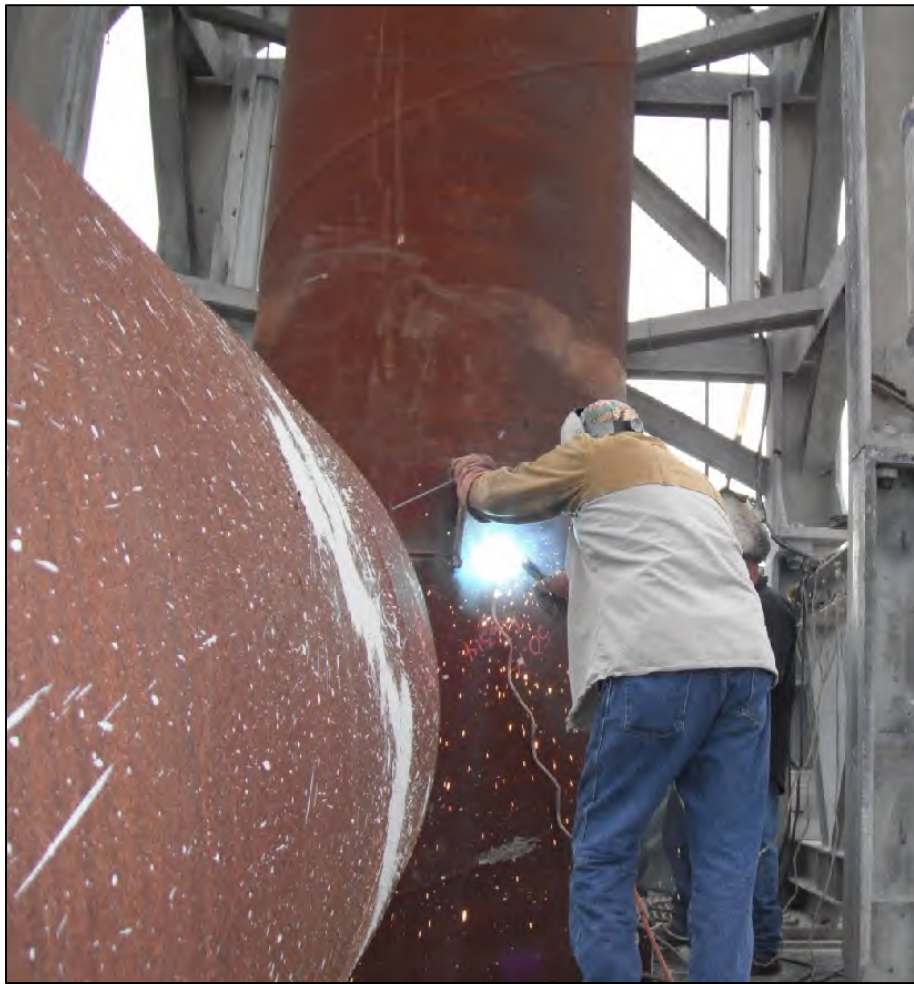
FIGURE 2-13 52-INCH SURFACE CASING INSTALLATION
