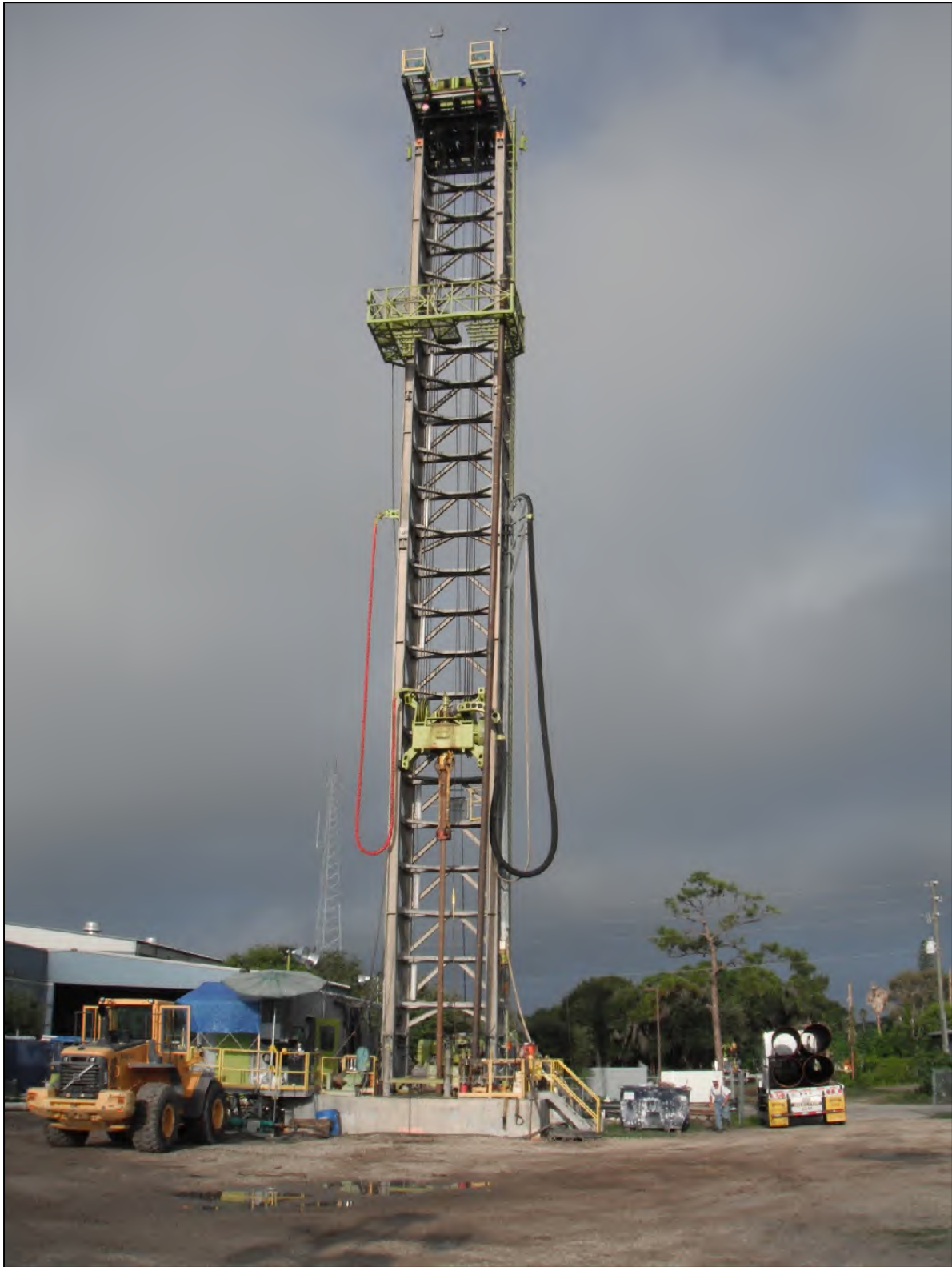
FIGURE 2-3 INJECTION WELL DRILLING RIG – YBI E2
