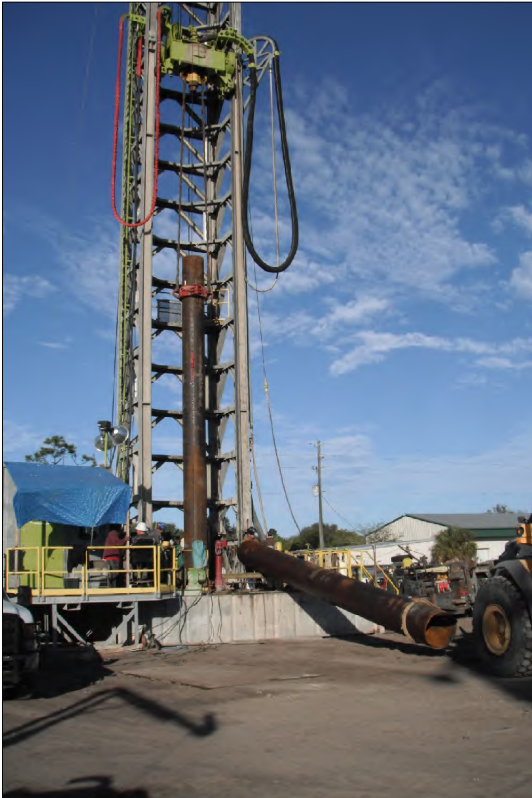
FIGURE 2-14 40-INCH DIW INTERMEDIATE CASING INSTALLATION
