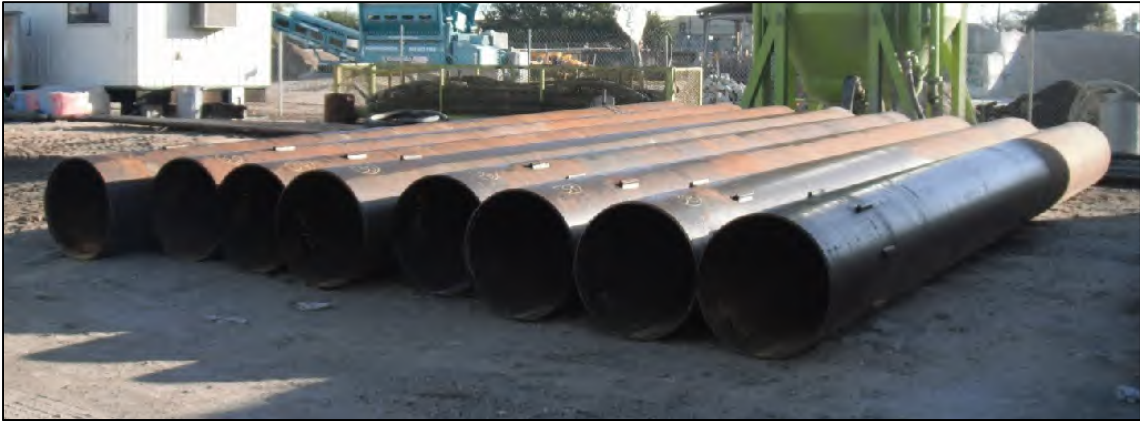
FIGURE 2-11: 28-INCH INJECTION WELL FINAL CASING
