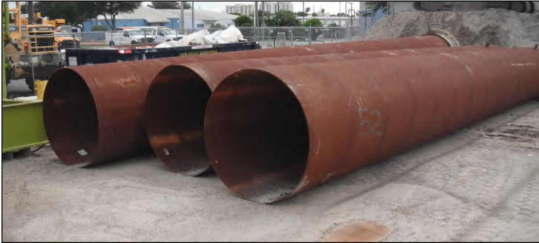
FIGURE 2-9: 52-INCH SURFACE CASING
