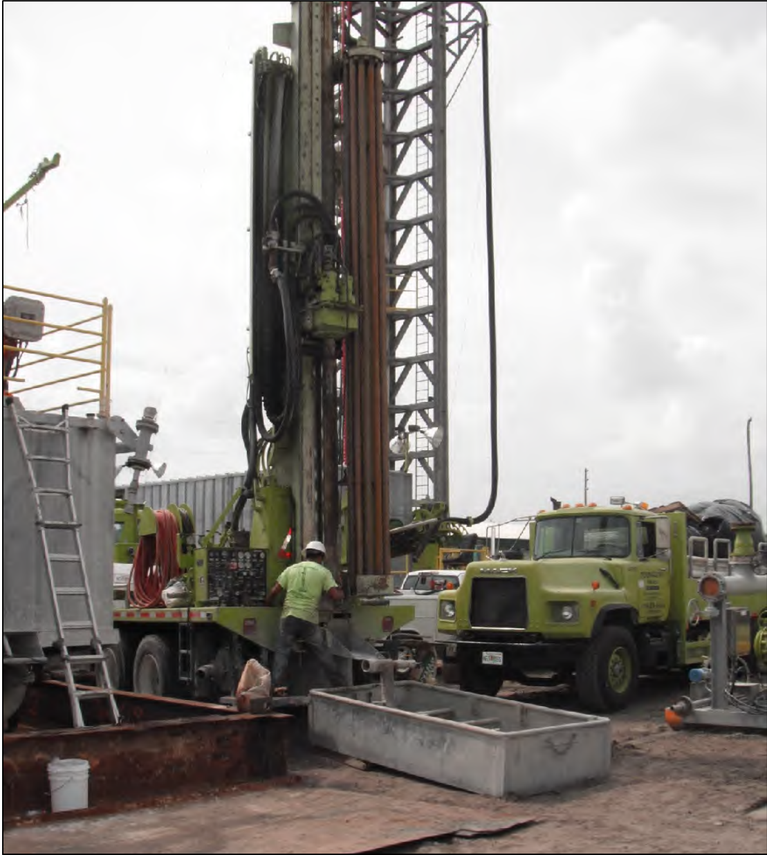
FIGURE 2-1 TRUCK MOUNTED DRILLING RIG FOR INSTALLATION OF SURFICIAL AQUIFER MONITOR WELLS
