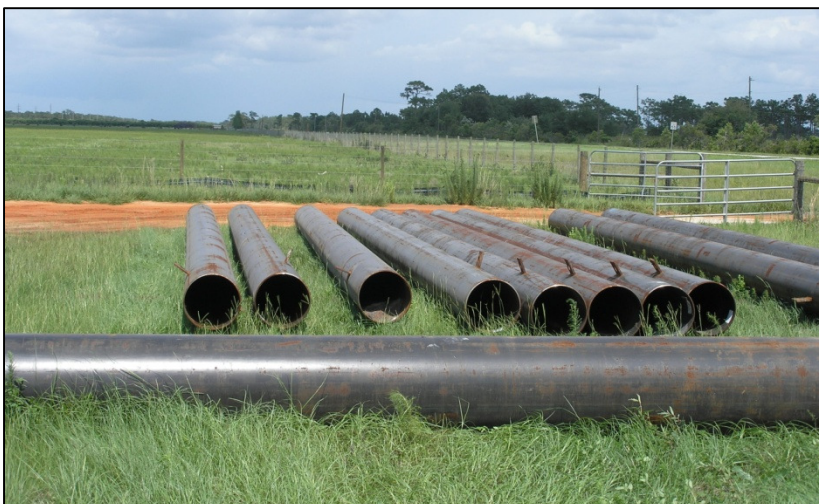
STEEL CASING : 14-INCH
