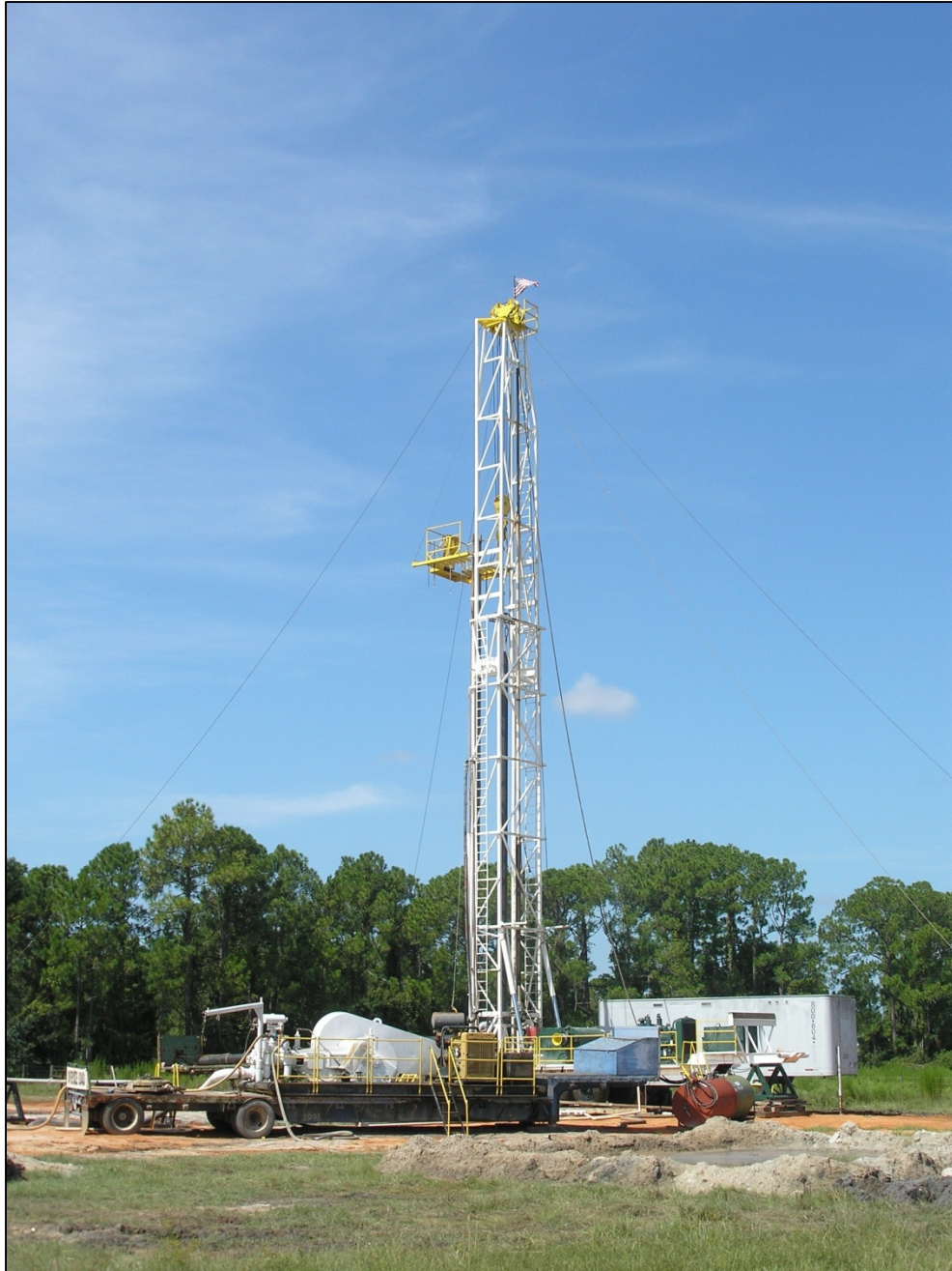
SE DZMW-1 DRILLING SITE & GARDNER DENVER 3000 DRILLING RIG
