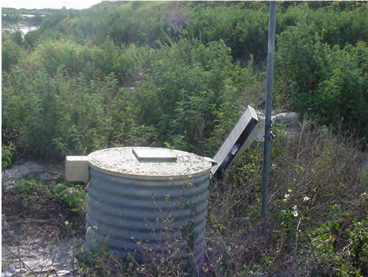
Pickett & Associates, Inc. Date of Survey: March 11, 2003 Looking: West
