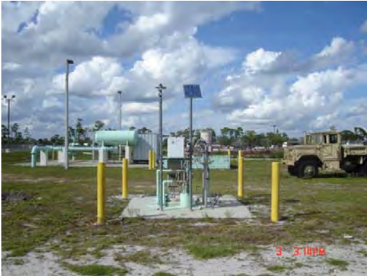
WELL AREA LOOKING NORTH
