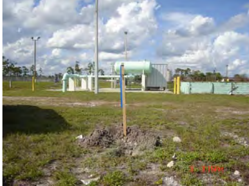
BENCHMARK AREA LOOKING NORTH
