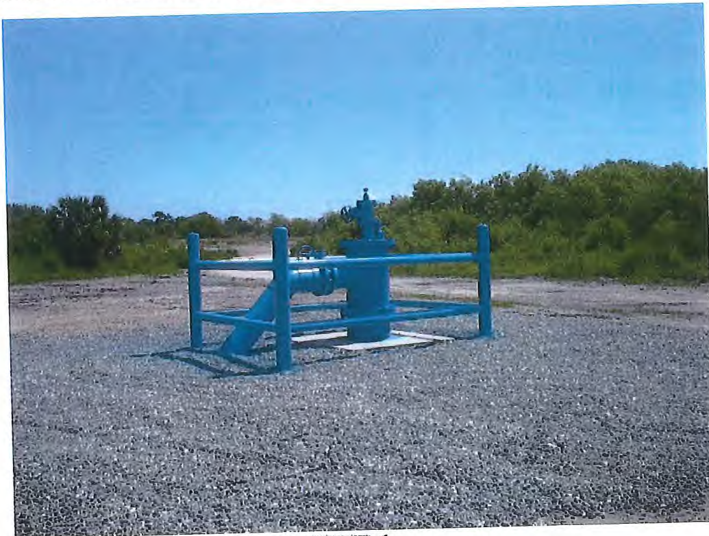
Figure 5. Completed Wellhead – EXKR-1
