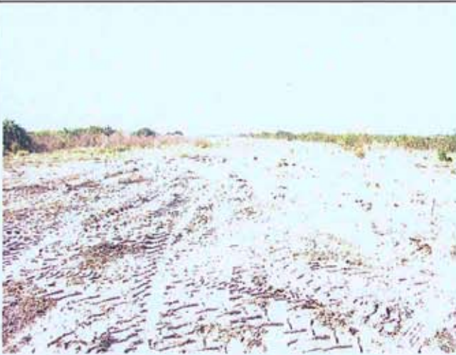
Photo 7: Previous location of well EXBRY-1 upon completion of plug and abandonment activities
