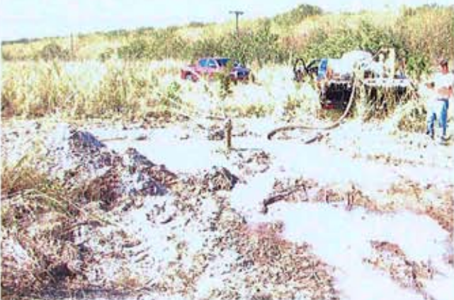
Photo 8: Cementing well CCBRY-1
