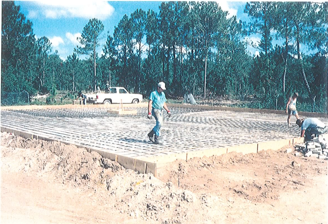
INJECTION WELL DRILL PAD UNDER CONSTRUCTION
