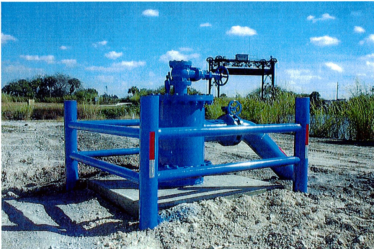
Figure 4. Completed Wellhead – Exploratory Well (EXPM-1).
