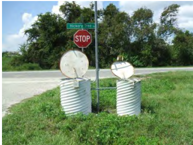
Sensor Well Area:
