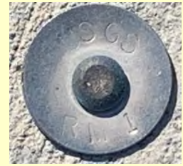
RM 1 – Nail in concrete curb inlet
