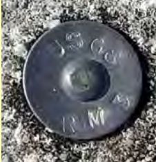
RM 3 – Nail in concrete utility slab
