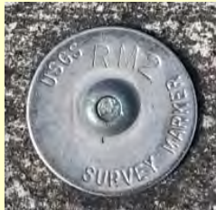
RM 2 – Nail and disc in concrete sidewalk
