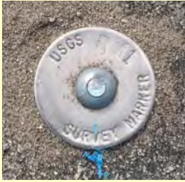
RM 1 – Nail and disc in concrete slab
