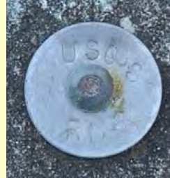
RM 2 – Nail and disc in concrete sidewalk
