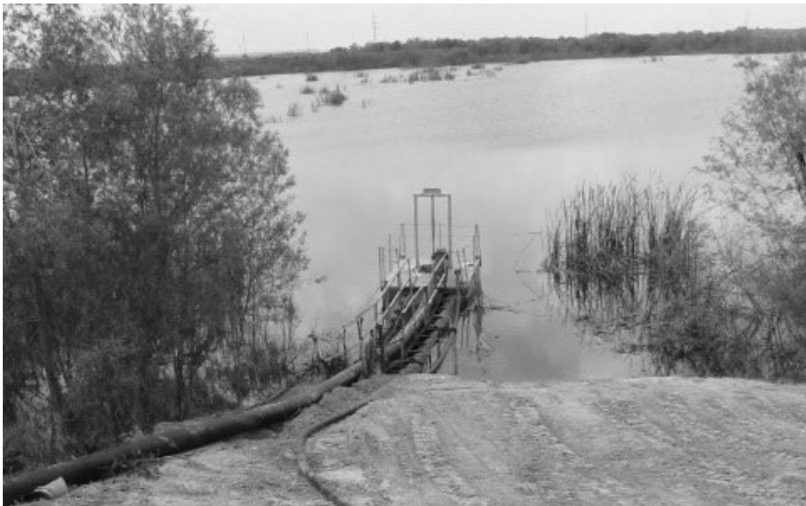
Figure C-6. SA-8 Pumping Station.
