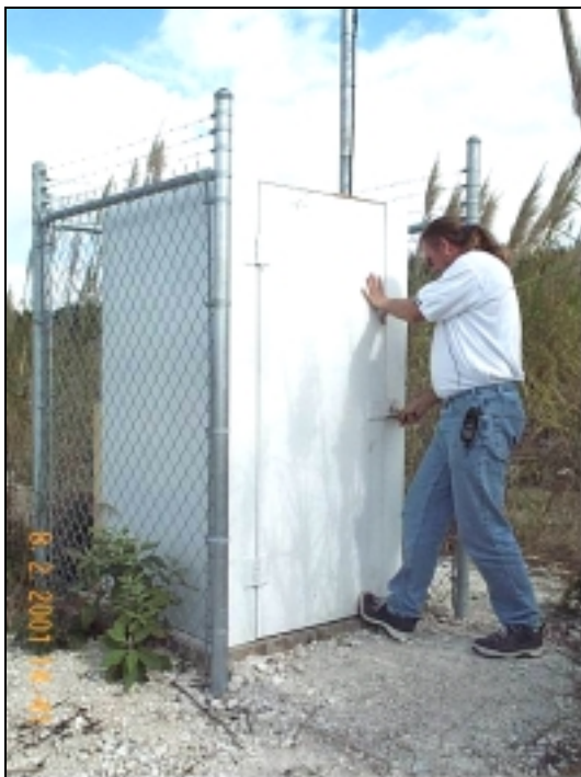
Figure 9. DF-3,4,5 Tri-Zone Monitor Well Enclosure.
