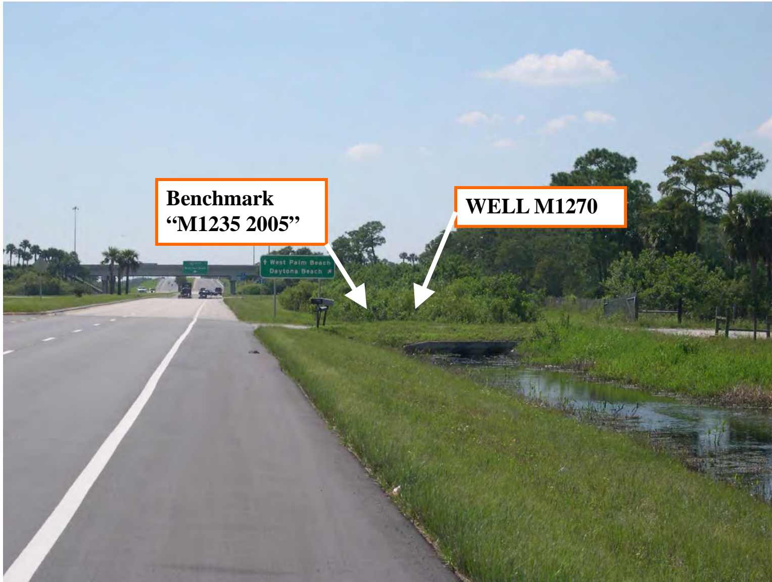
Biscayne Engineering Company, Inc. Date of Photo: 09-12-05 View: Looking West along Bridge Road (SR 706) at I-95 (Well location near driveway at right)
