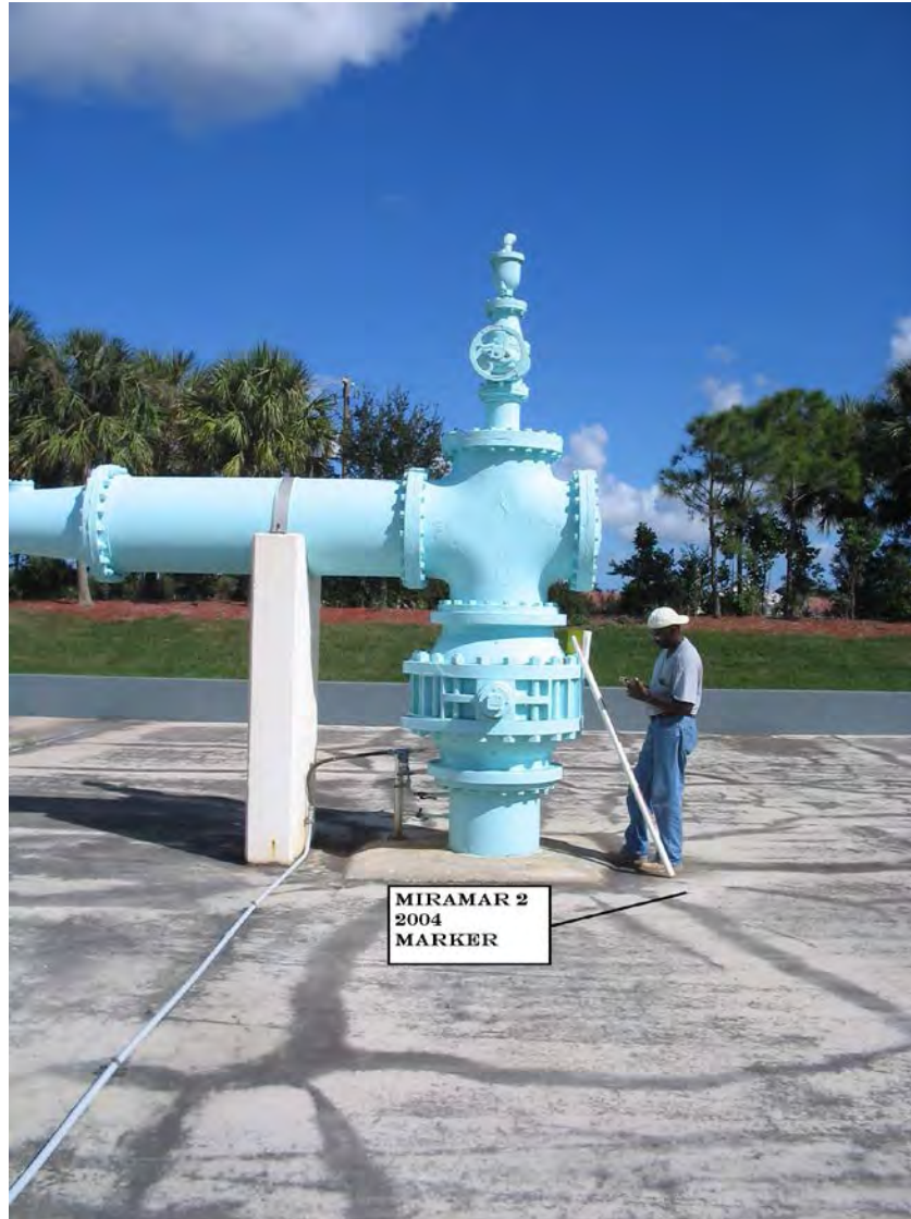
Biscayne Engineering Company, Inc. Date of Photo: 11-03-04 View: Looking East
