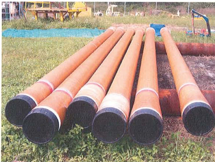
10.75-inch nominal Fiberglass Reinforced Plastic tubing on site ready for installation
