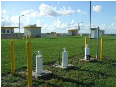
Sensor Well Area:
