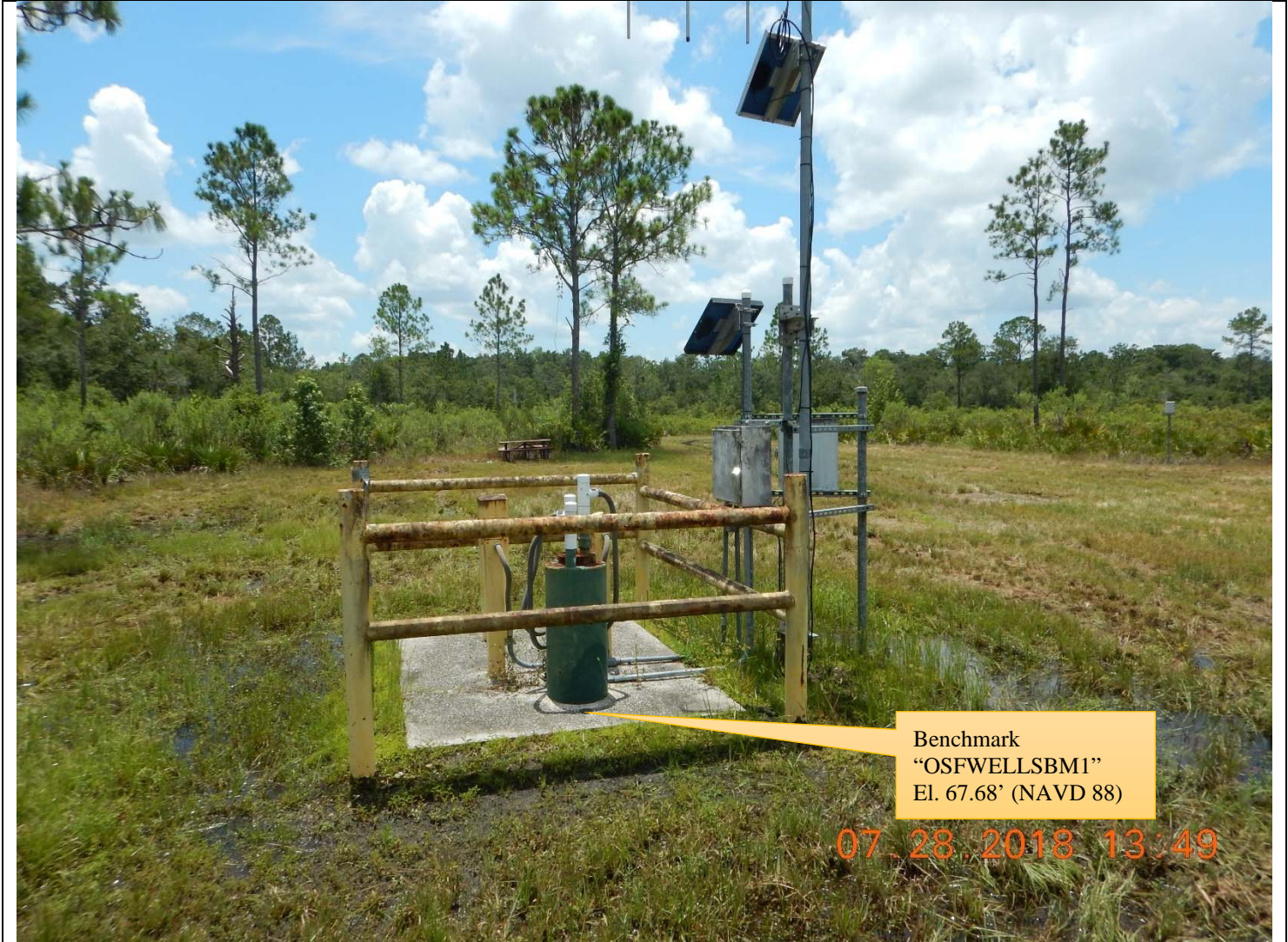
Looking West (Oblique not to scale) (July 28, 2018)
