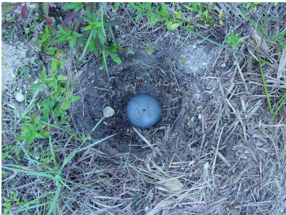
View: Close-up of the well PB 1632 showing the contractor's markings
