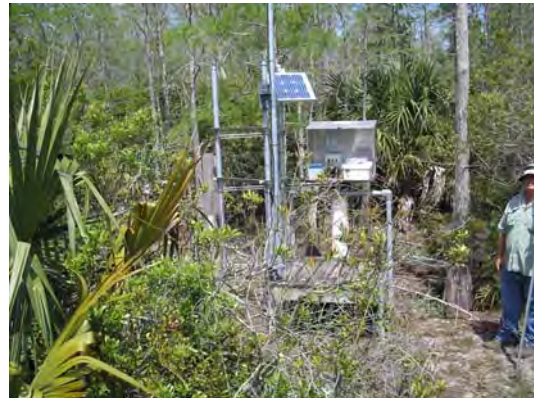
STG1 AREA LOOKING NORTH
