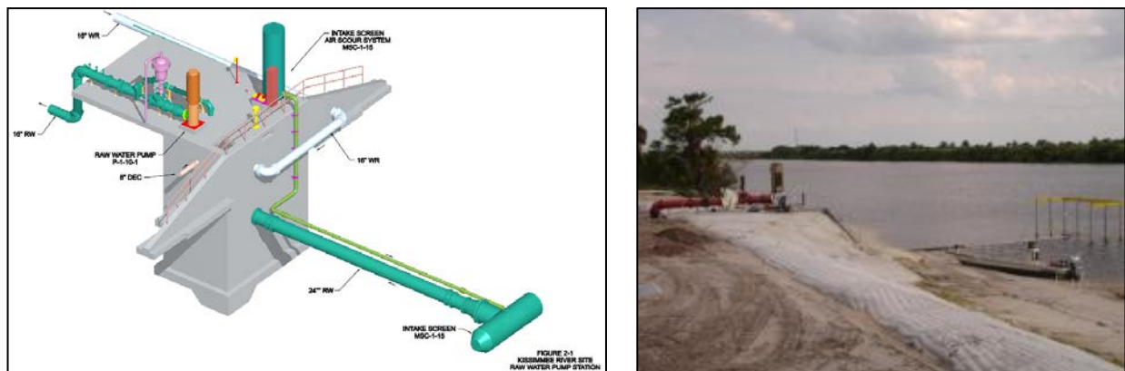
Figure 6-2 -- Intake design layout (left), and intake structure under construction (right).
