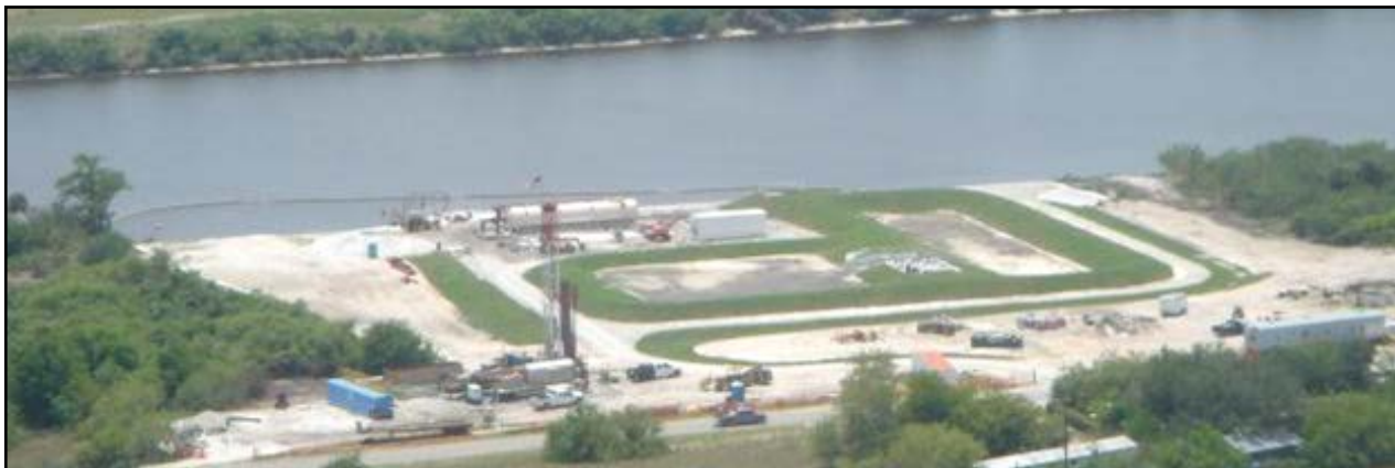
E. ASR system construction in progress – June 2007. Drill rig in lower left is constructing the 350-ft SZMW.
