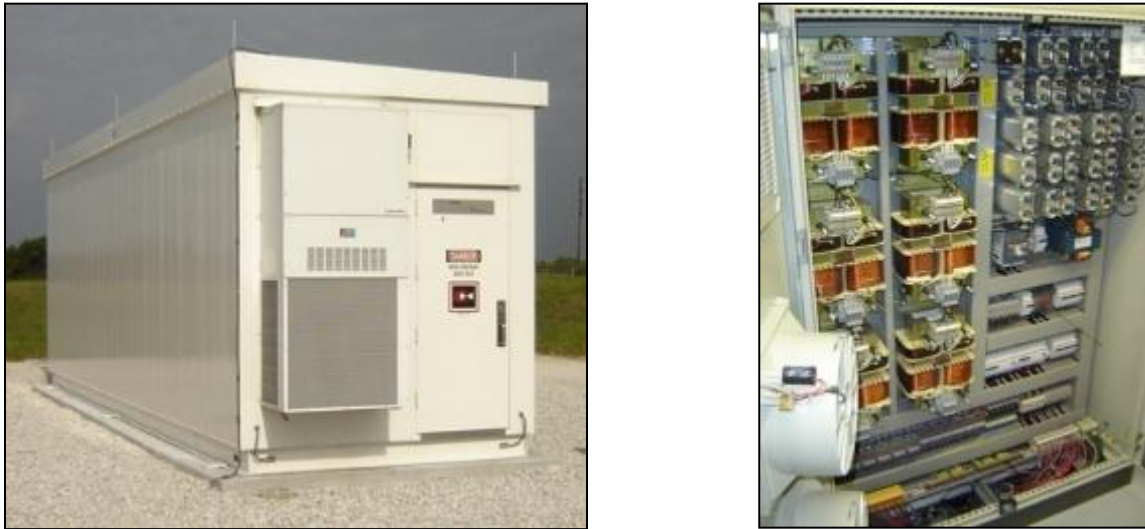
Figure 6-12 -- The electrical and motor control center enclosure (left); and UV disinfection system control unit box (right).
