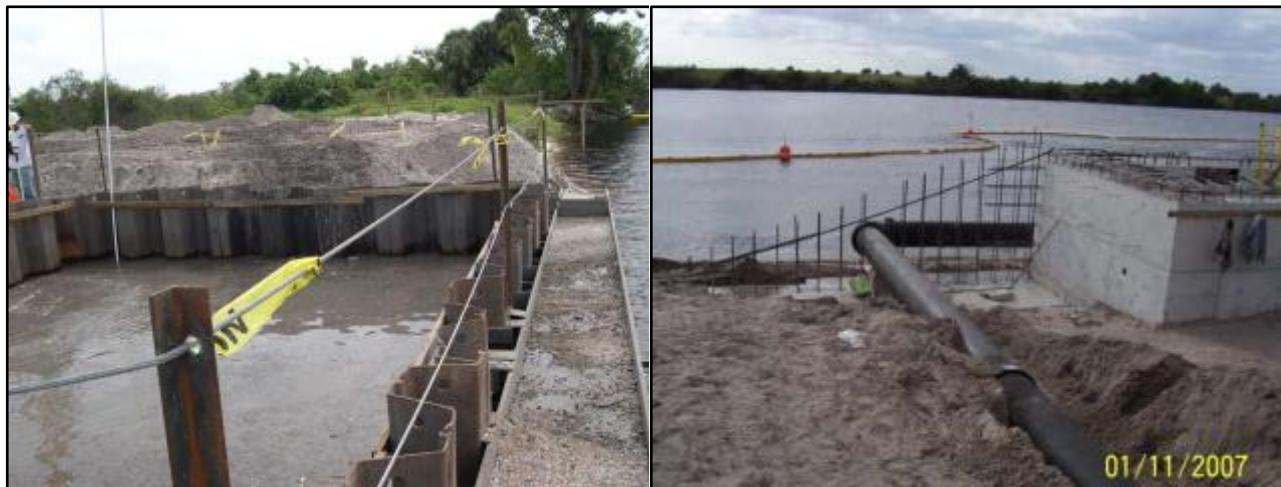
A. Cofferdam for wet well construction. inlet pipe.
