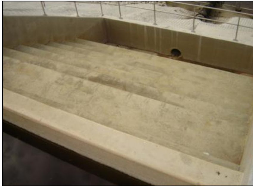
Figure 6-10 -- The spill structure and cascade aerator.
