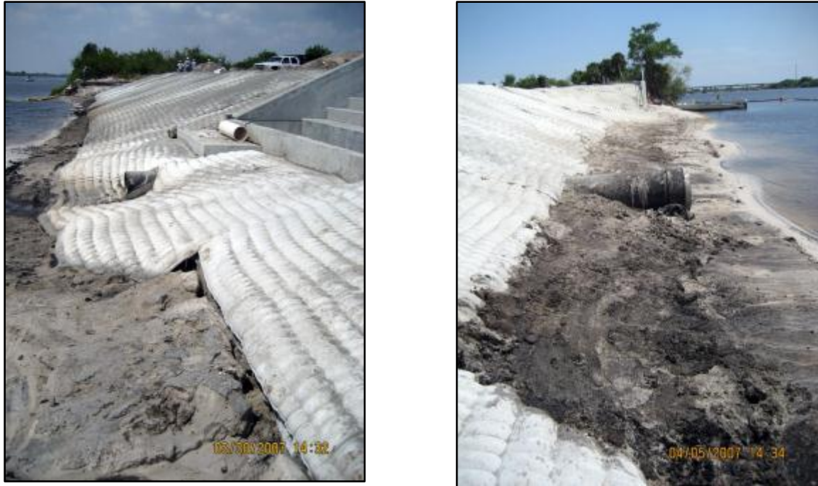
Figure 8-4 -- Embankment erosion control before (left) and after (right).
