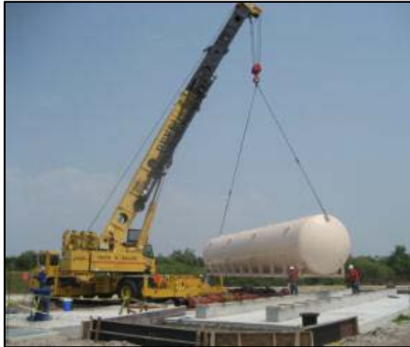
C. Installing the pressure filter.
