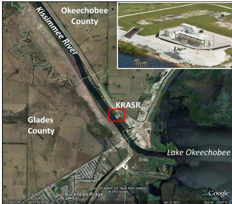
Figure 3-3 -- Location of the Kissimmee River ASR (KRASR) system. Inset is an aerial view of the ASR system.
