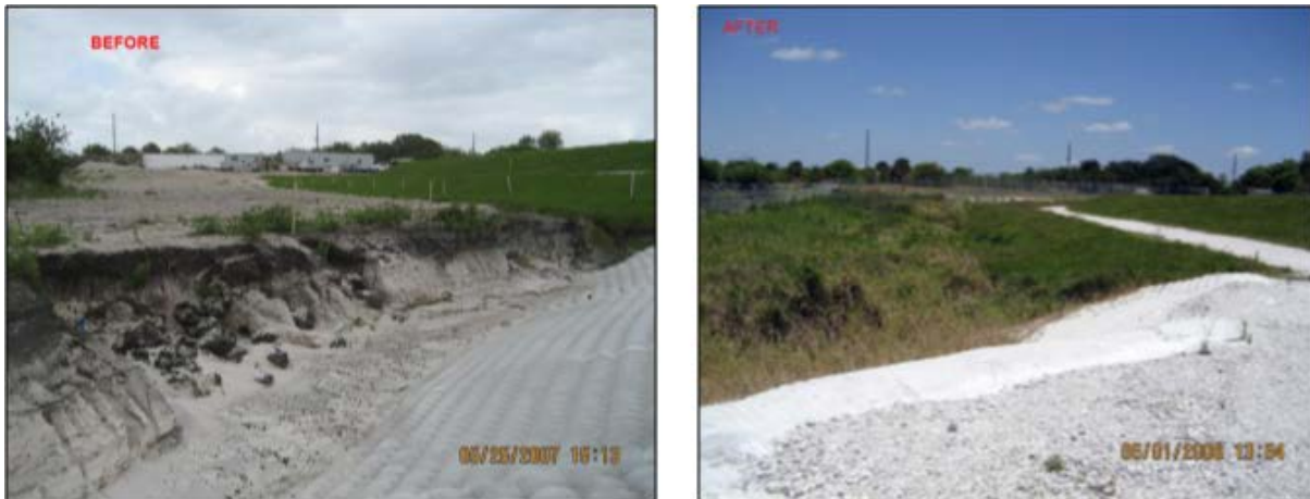
Figure 8-5 -- Erosion control along drainage swales, before (left) and after (right).
