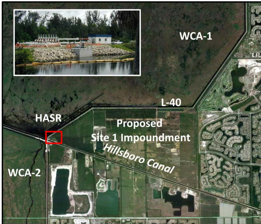
Figure 3-4 -- Location of the Hillsboro ASR (HASR) system. Inset is a panoramic view of the ASR system.
