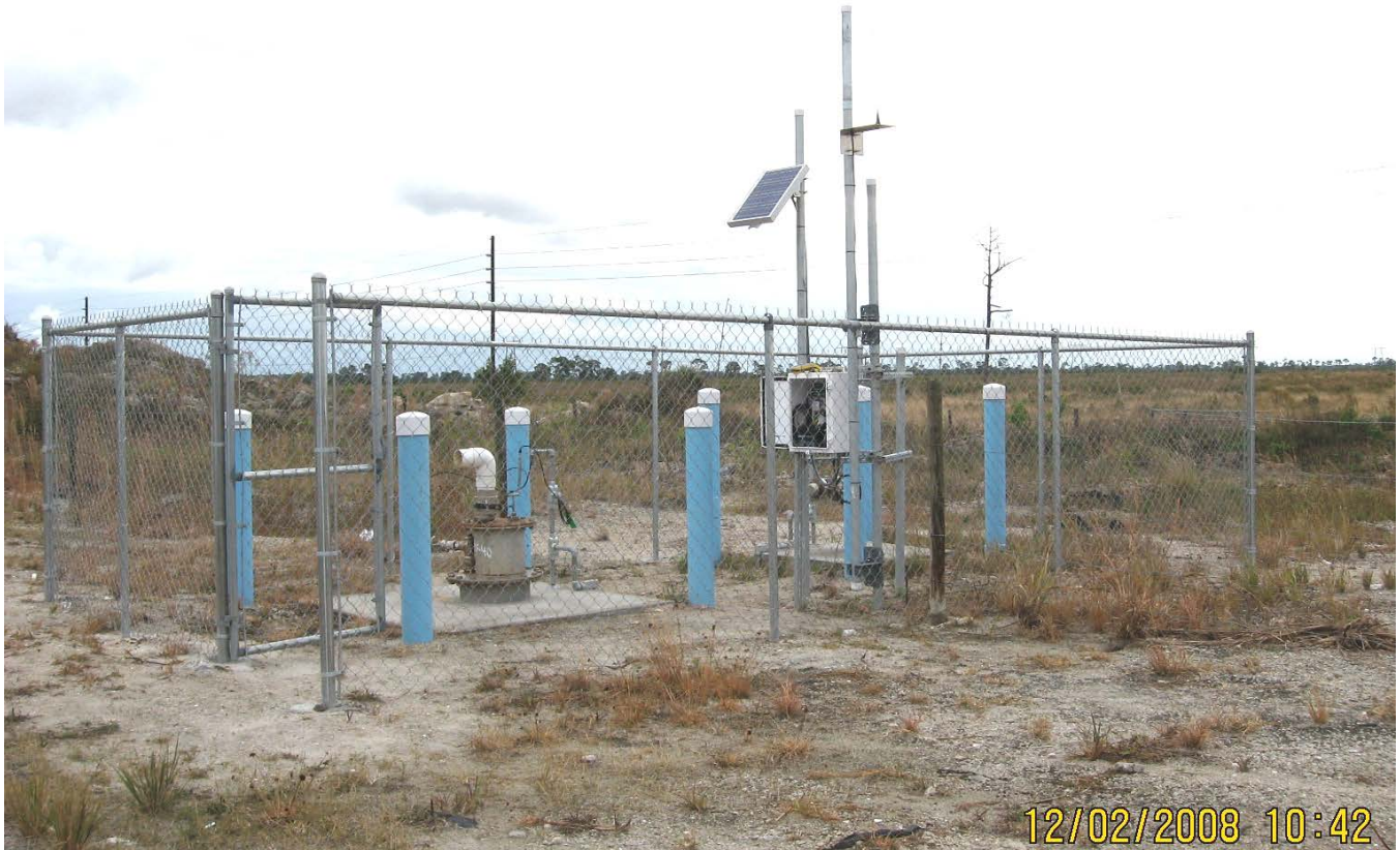
Looking Southeast (District Picture 02-dec-08)
