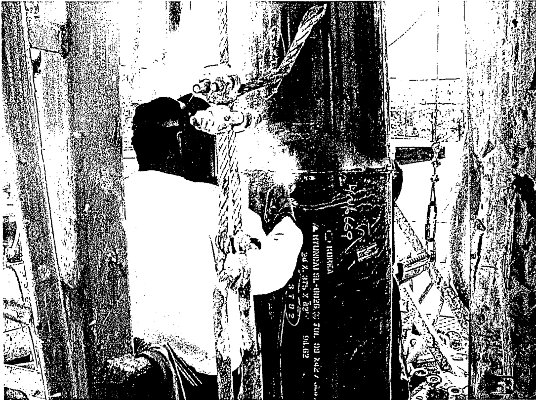
FIGURE 2-7 Welding Sections of 24-inch Casing
