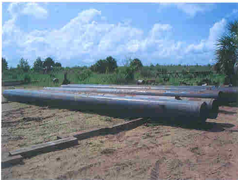
Photograph D-6- 24-inch casing
