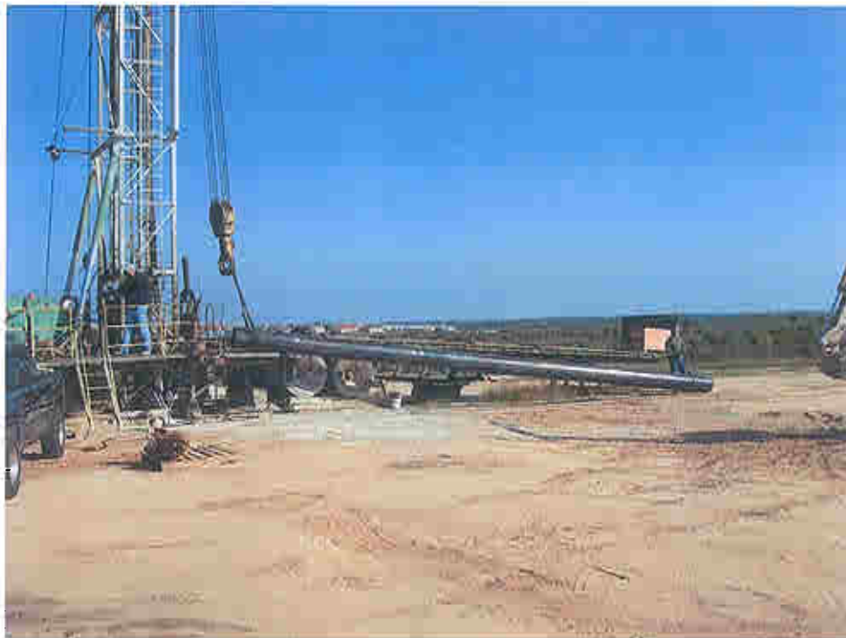
Photograph D-10 - 18-inch steel casing
