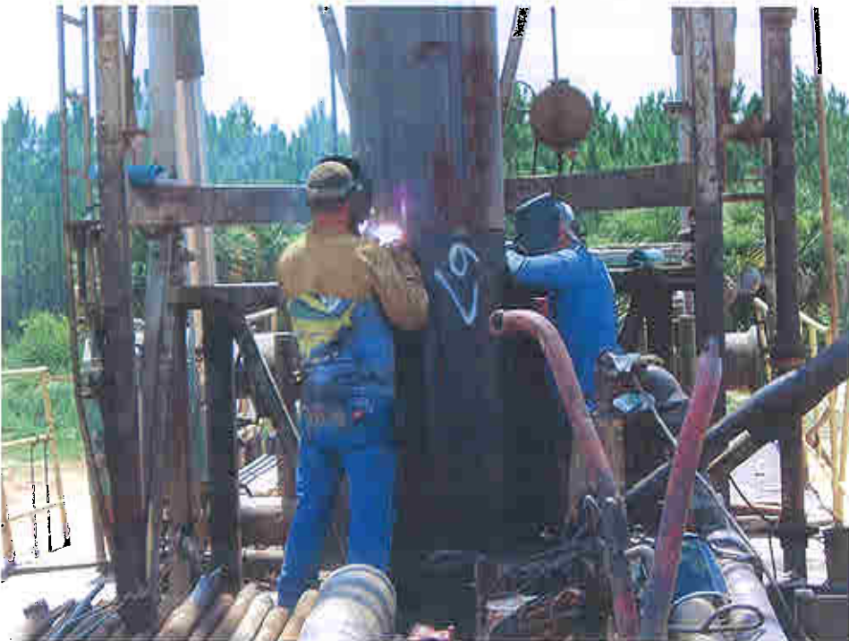
Photograph D-8 - Welding 24-inch casing
