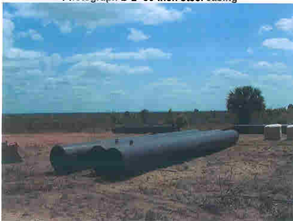
Photograph D-2- 36-inch steel casing
