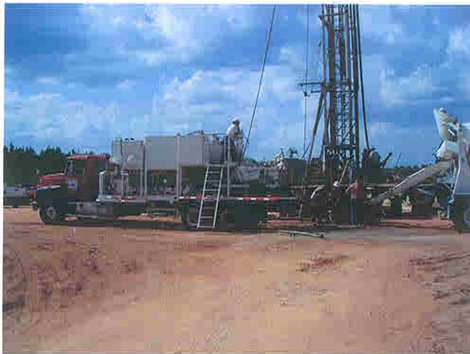
Photograph D-5- Cementing Operation
