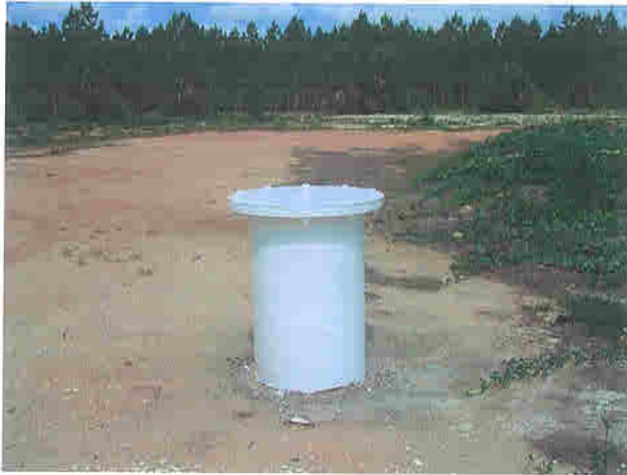
Photograph D-19 - HH-1 Wellhead Completion
