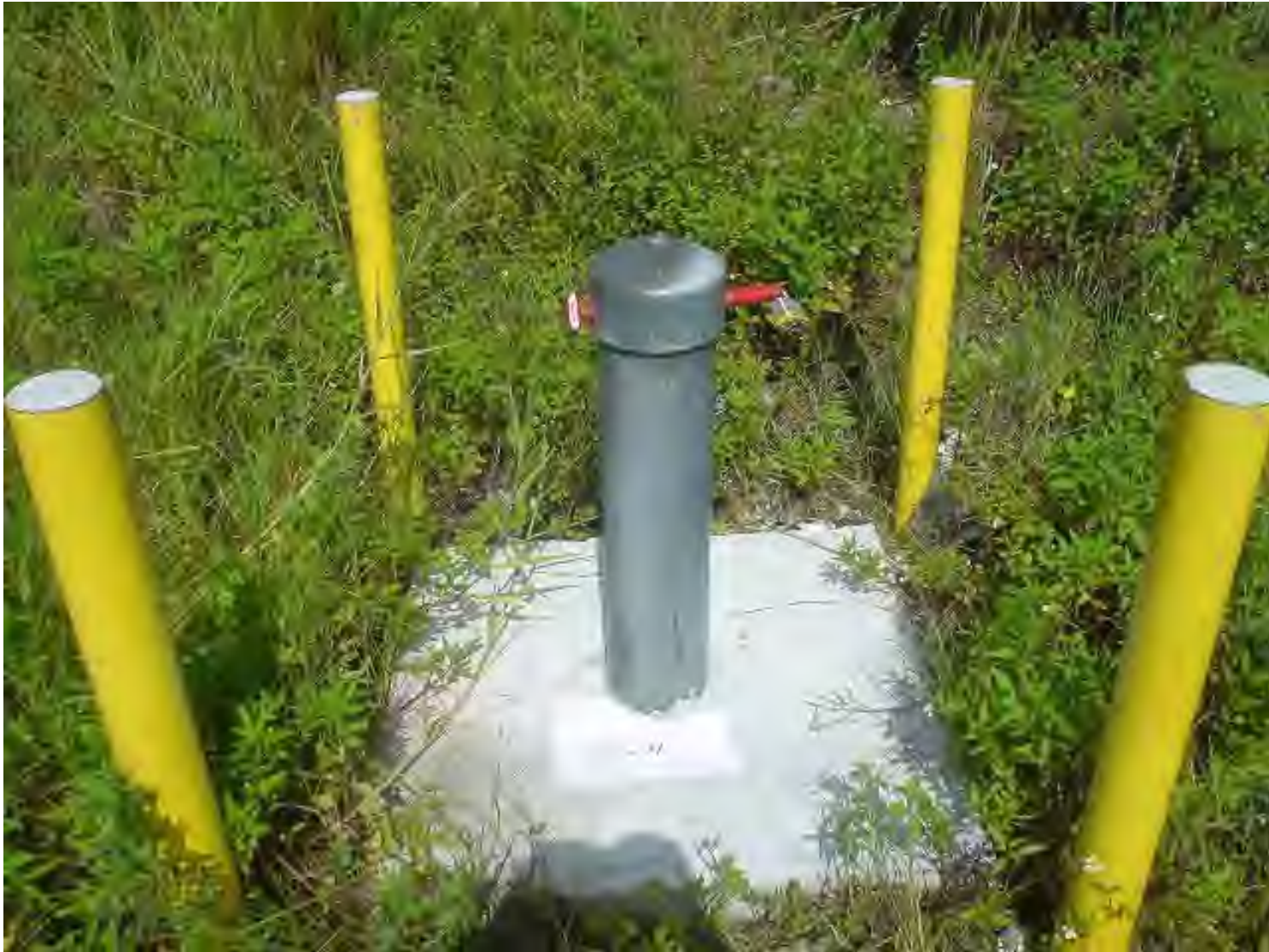
Weidener Surveying & Mapping, P.A. Date of Photo: July 21, 2005 View: Geotechnical Well
